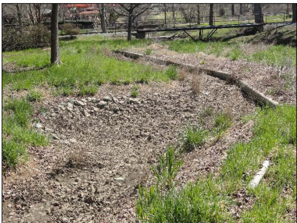
Photo Station 2, level spreader at bollard 410, facing east: April 3, 2013
