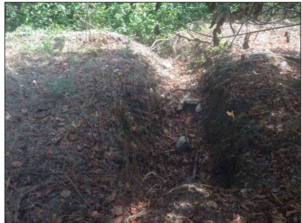
Photo Station 4, discharge at bollard 312, facing west: September 3, 2015
