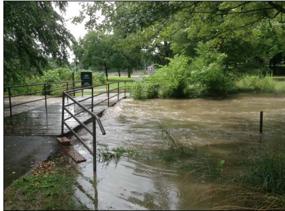
Bridge at XS 5 July 3, 2013
