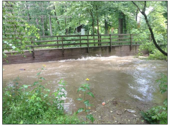
View of Bridge at XS 4 July 3, 2013
