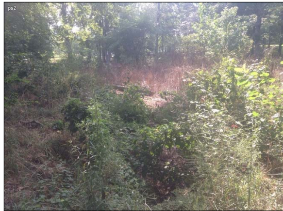
Photo Station 2, level spreader at bollard 410, facing east: September 3, 2015
