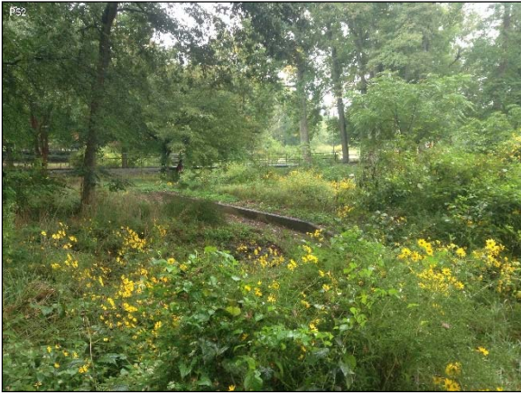
Photo Station 2, level spreader at bollard 410, facing east: September 30, 2014
