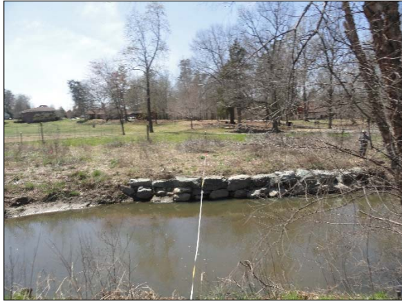
Photo Station 13, XS 7, facing right bank: April 3, 2013
