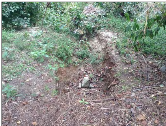
Photo Station 4, discharge at bollard 312, facing west: October 5, 2016
