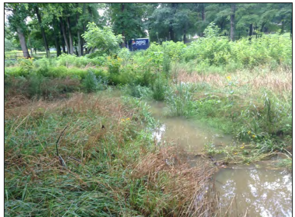
View from PS 2, level spreader July 3, 2013
