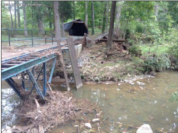
Wreck line and debris from flooding including a picnic table at the train bridge closest to VP5.
