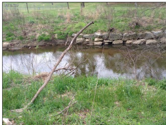
Photo Station 13, XS 7, facing right bank: March 31, 2016
