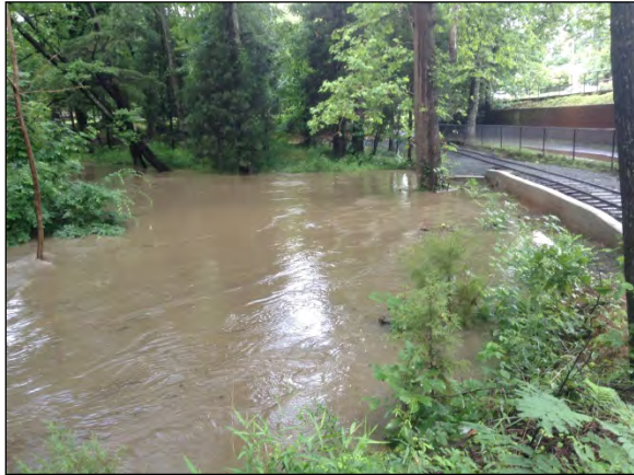
View of Rail Road at PS1 July 3, 2013
