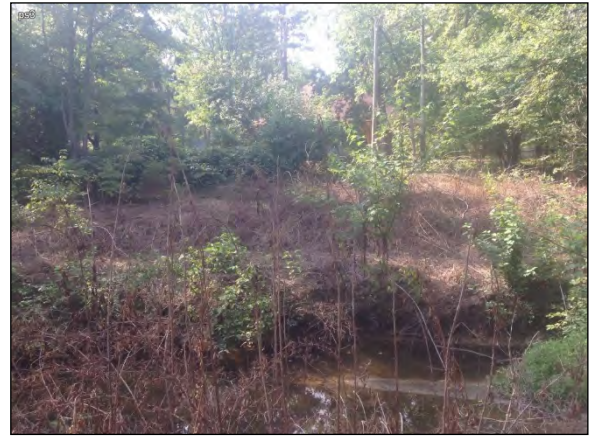
Photo Station 3, rail line discharge, facing south: September 3, 2015
