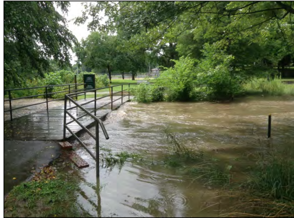
Bridge at XS 5 July 3, 2013
