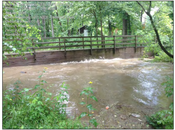
View of Bridge at XS 4 July 3, 2013
