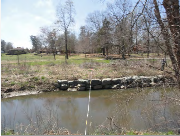
Photo Station 13, XS 7, facing right bank: April 3, 2013
