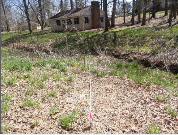
Photo Station 19, XS 13, facing right bank: April 3, 2013
