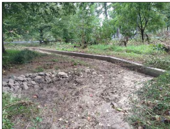
Photo Station 2, level spreader at bollard 410, facing east: October 5, 2016
