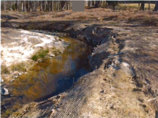
VPA 23. Vegetation not establishing through coir matting.
