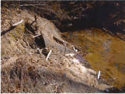
VPA 1. Unvegetated coir matting on both banks.
