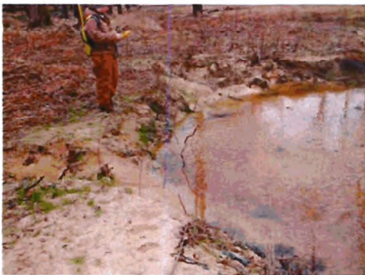
SPA 17. Aggradation in pool. Sta. 26+78.
