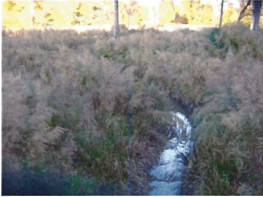
Photo Point 24. Facing upstream from culvert at end of project.
