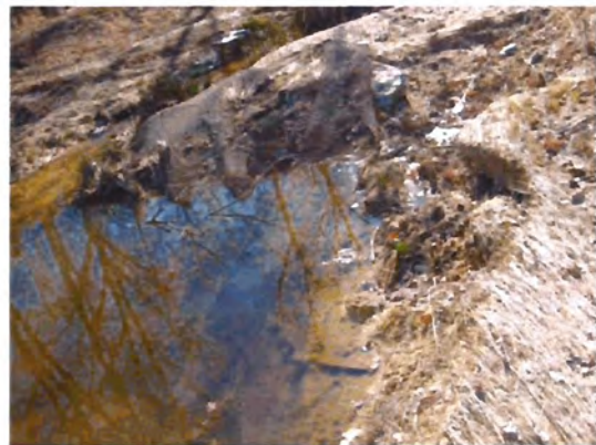
VPA 12. Vegetation not establishing through coir matting.
