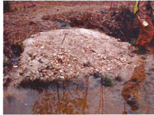
SPA 6. Deposition in mid point of curve. Sta. 15+27.
