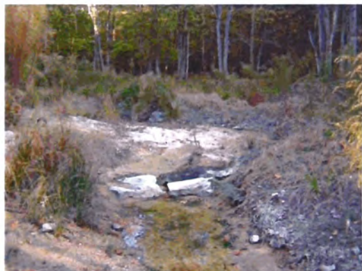
Photo Point 13. Facing upstream from sill.
