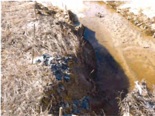
VPA 20. Vegetation not establishing through coir matting on both banks.
