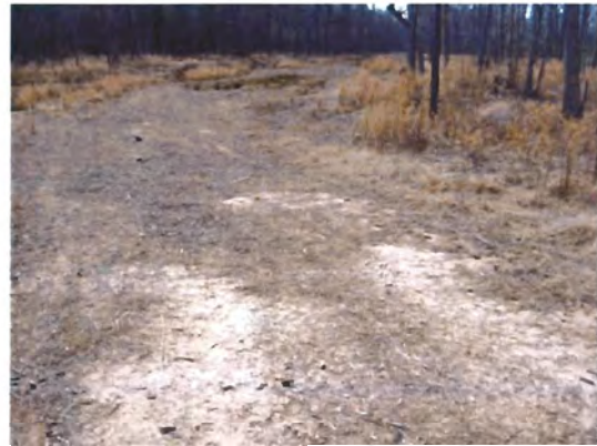
VPA 5. Dirt road through overly mulched area.
