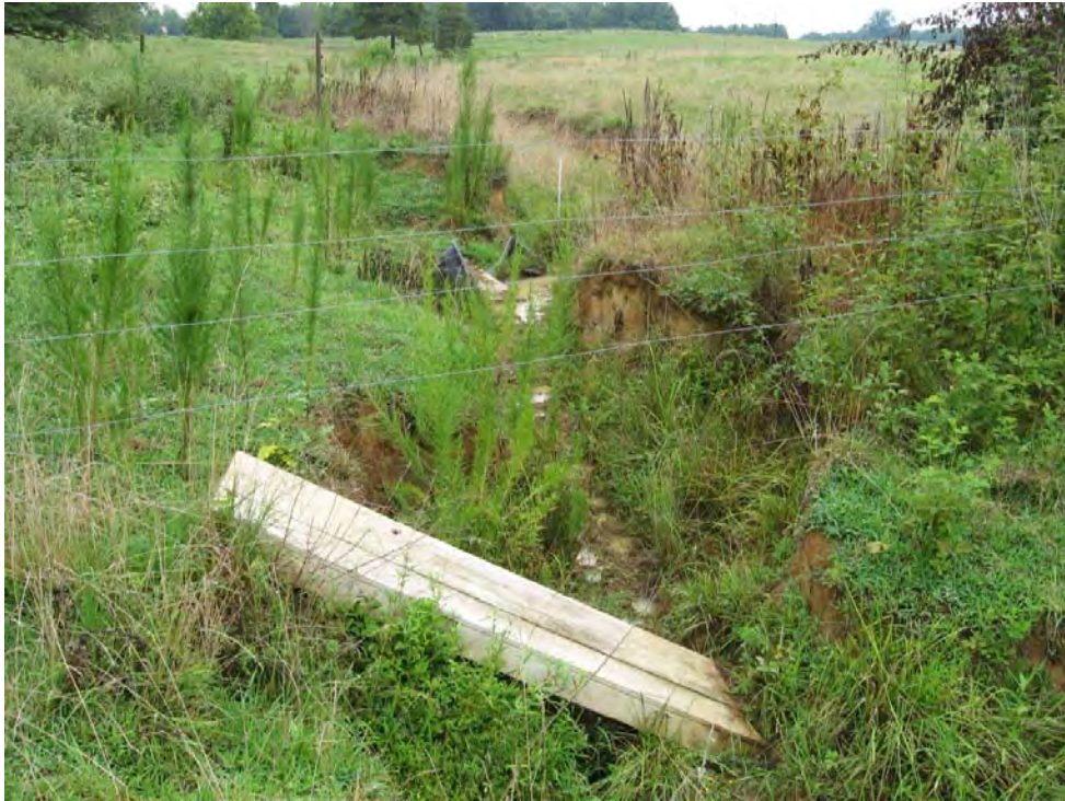
Photo 13: UT 3. View looking upstream at E-1 area. (7/27/2010)
