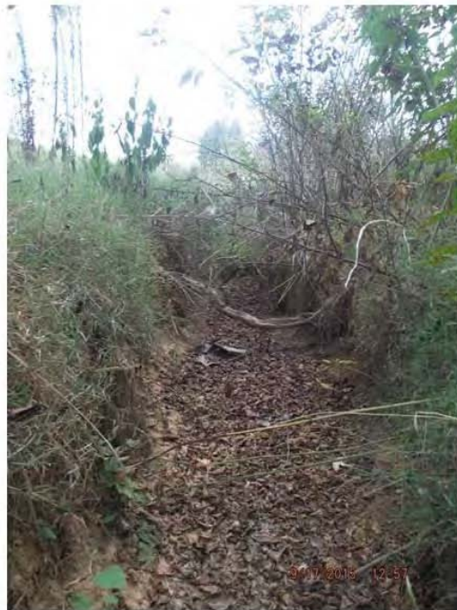
Reach 4 - Head cut in UT3 upstream of gage 7
