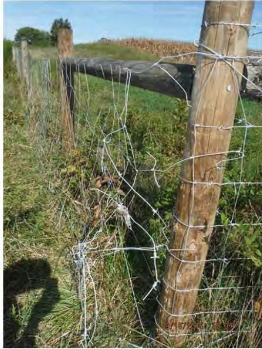
Reach 4 - Fence cut, baro-logger missing
