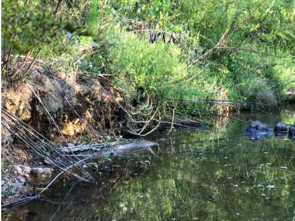
Undercut along the left interior channel bank in restoration area of reach 3
