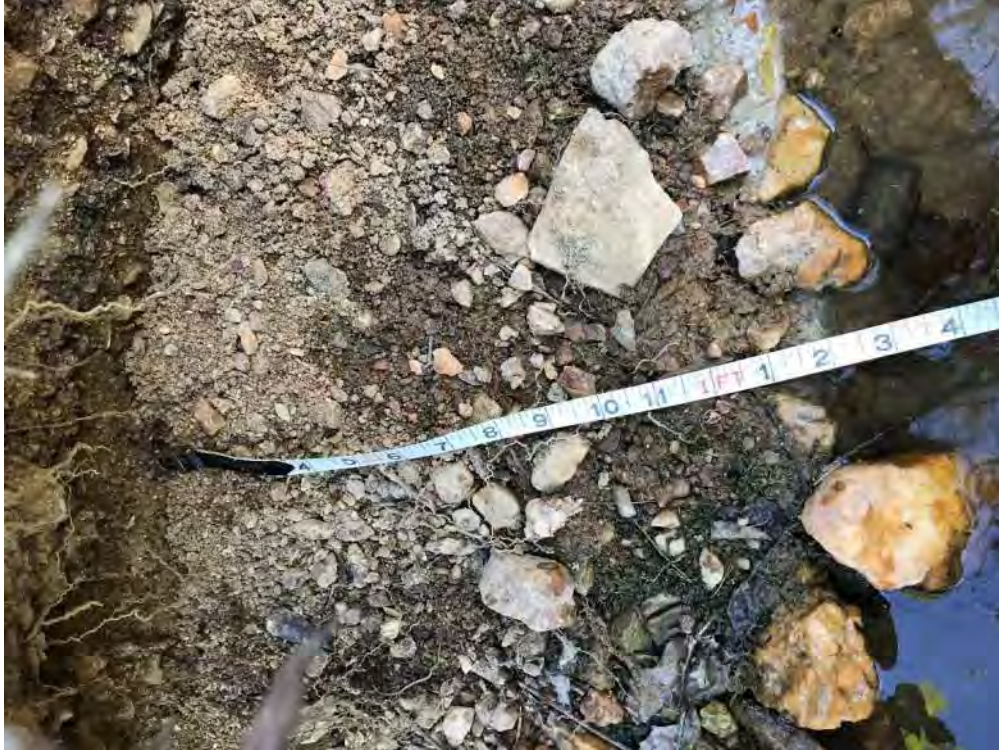
Undercut along the left interior channel bank in restoration area of reach 3
