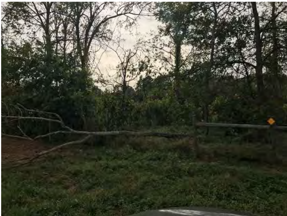
Tree fallen on easement fence at UT7. Minor damage will need repair.
