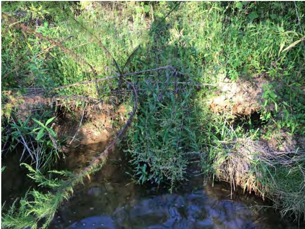
Undercut along the left interior channel bank in restoration area of reach 3
