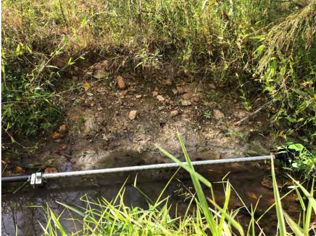
6 foot bank scour along the right bank in restoration area of reach 4
