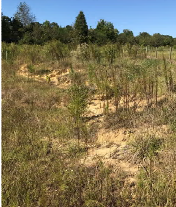
Bare spots and eroding slopes on outskirts of floodplain in reach 1
