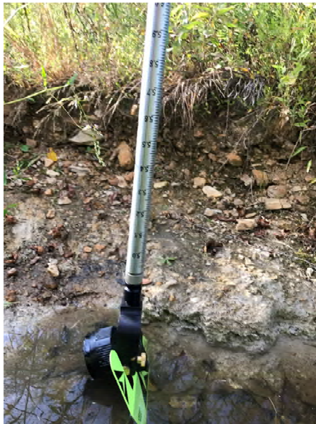
6 foot bank scour along the right bank in restoration area of reach 4
