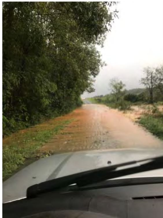
Flooding over old mine road at UT7
