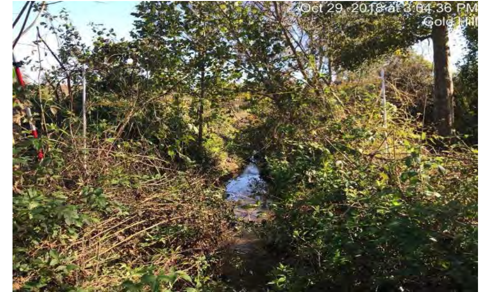
1391.34 UT2-1R Looking Downstream
