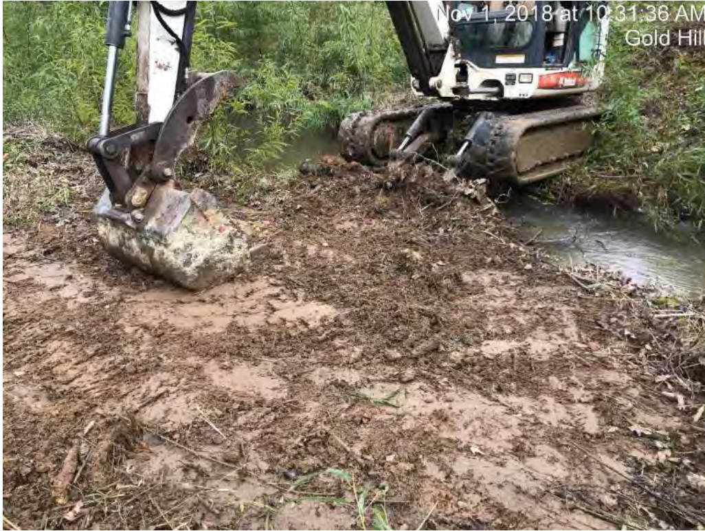
Beaver dam removal from Reach 1 (during project)
