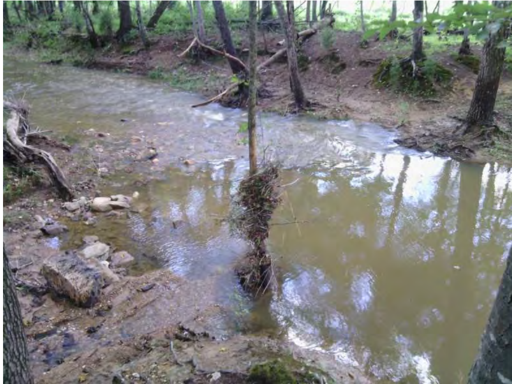
Wrack line indicating high water levels Photo take in September 2018
