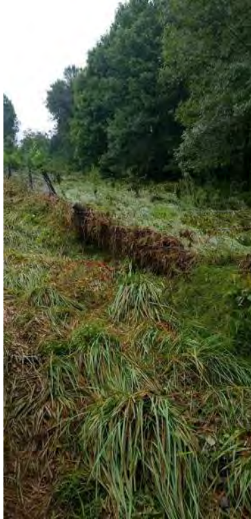
Bent vegetation into easement fence from hurricane
