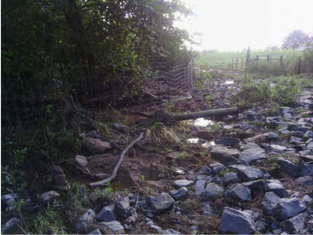
Blown out cattle crossing (Reach 5)
