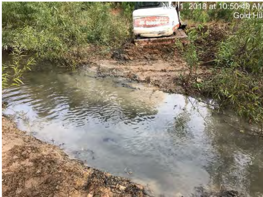
Beaver dam removal from Reach 1 (after removal)
