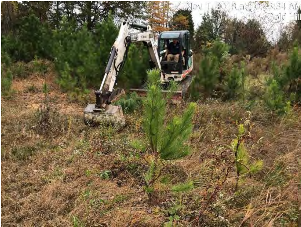
Beaver dam removal from Reach 1 (beginning)
