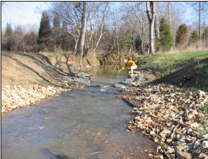
Cross vane on Little Grassy Creek during final walk-through
