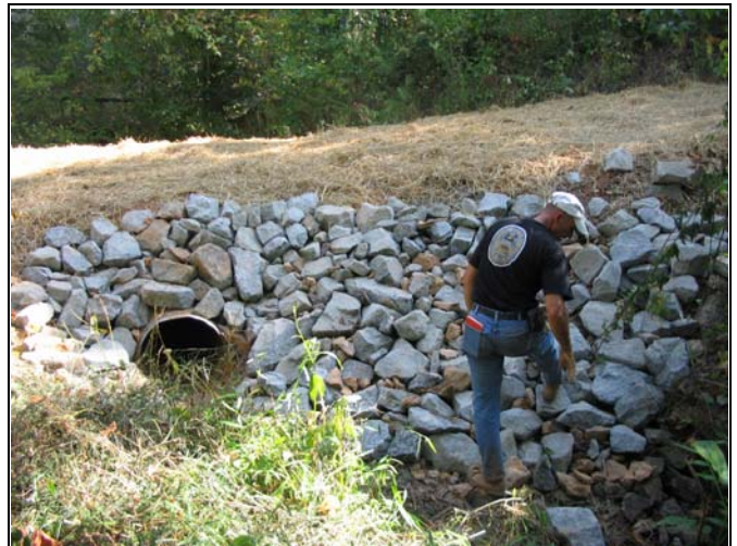
Culvert crossing stabilization
