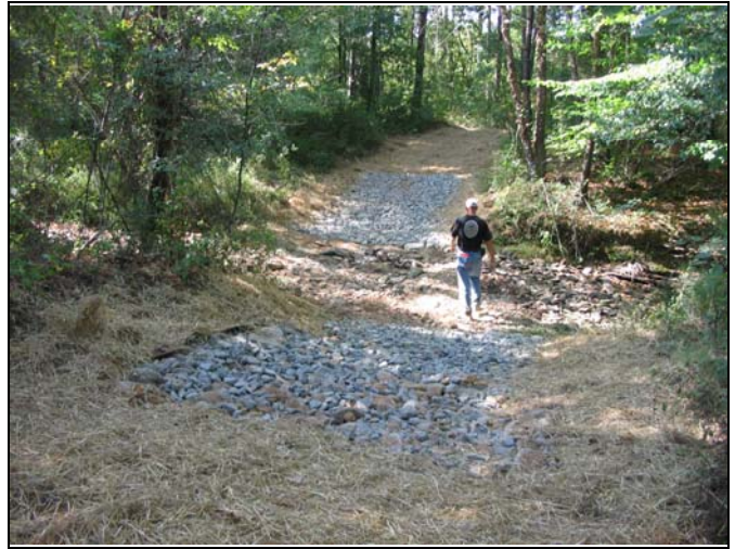
Ford crossing near the mill on Little Grassy Creek
