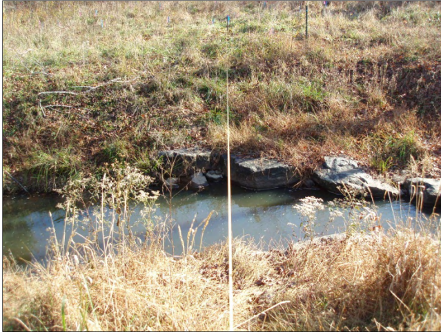
Cross-Section 4 – Looking across the stream at the right bank. 11/9/09 - MY 02
