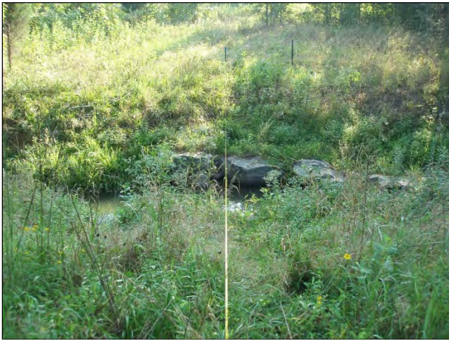
Cross-Section 4 – Looking across the stream at the right bank. 8/27/09 - MY 02
