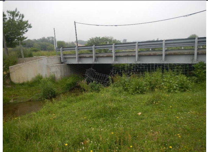
Glade Creek School Road bridge over Little Pine Creek, looking upstream.
