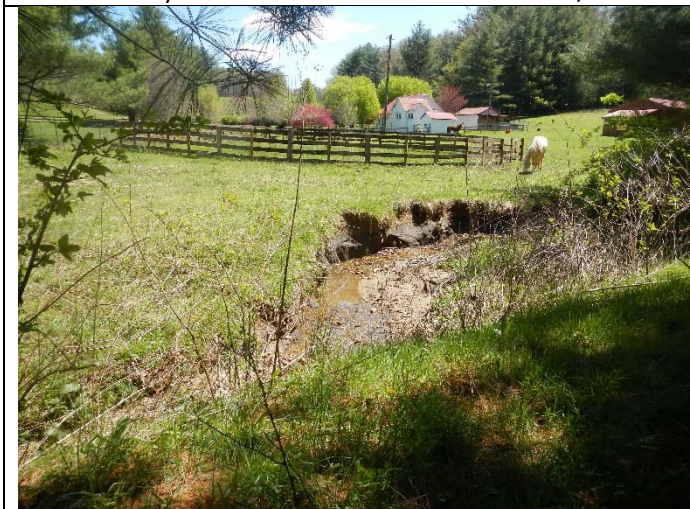
Looking upstream along Tributary C. 04/2015
