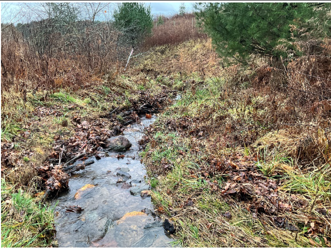
UT2A STA 426+50 – Phase III right and left banks repaired, looking downstream (12/7/2022)
