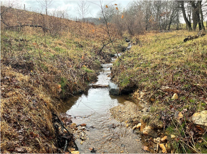
UT2 Reach 1 (Upper) STA 309+50 – 310+50 – Phase III rock cross vanes added, structures and left bank repaired, looking upstream (12/7/2022)
