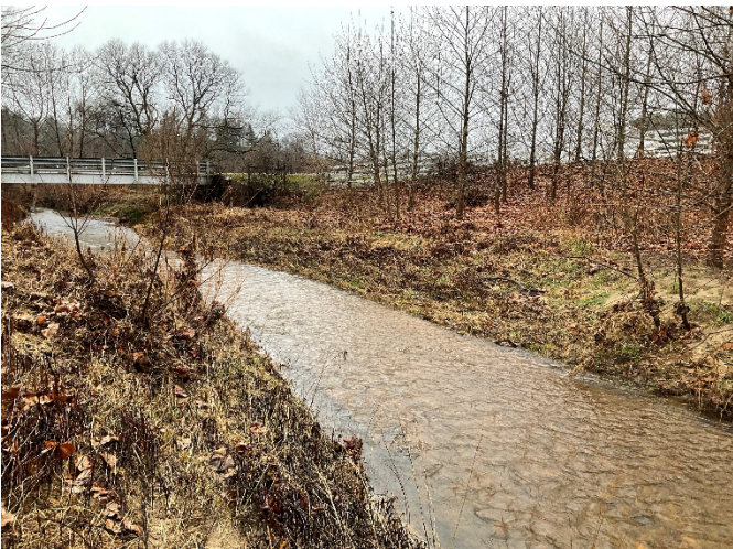
LPC Reach 2b STA 133+50 – Phase III right bank repaired, looking downstream (12/7/2022)
