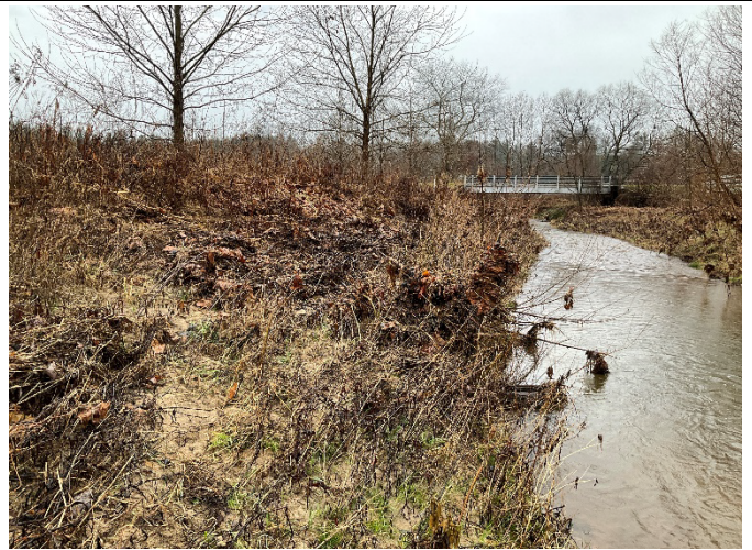
LPC Reach 2b STA 133+00 – Phase III left bank repaired, looking downstream (12/7/2022)
