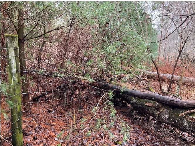
Conservation Easement Boundary – Located south of PP31 on UT2B, tree down on fence line, looking southwest (12/7/2022)
