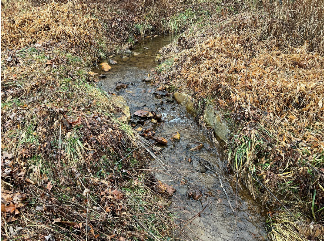
UT2 Reach 2 STA 330+00 – Phase III rock cross vane added, looking upstream (12/7/2022)
