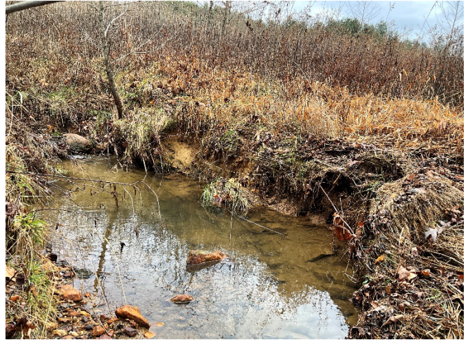
UT2 Reach 2 STA 336+40 – Left bank scour, looking upstream (12/7/2022)
