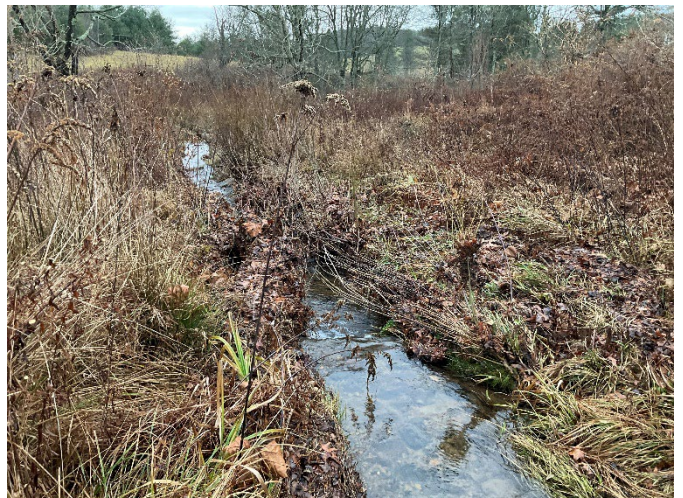
UT2A STA 431+60 – Phase I right bank repair area, looking downstream (12/7/2022)
