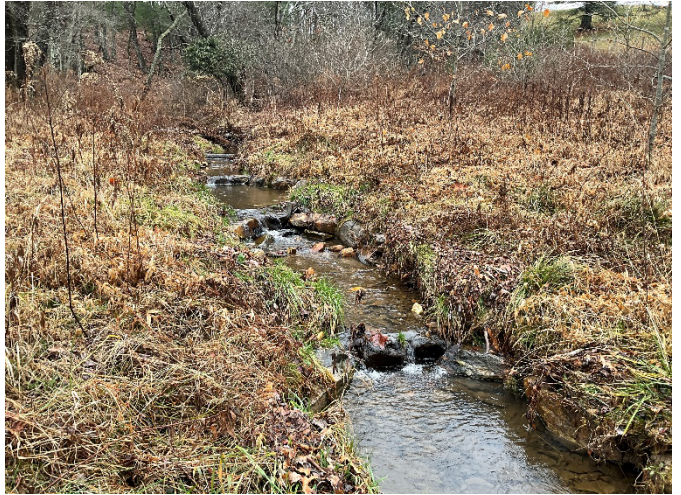
UT2 Reach 1 (Lower) STA 325+50 – 326+00 – Phase III buried channel rebuilt, rock cross vanes and riffles added, looking upstream (12/7/2022)
