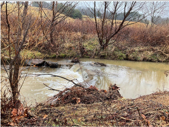
LPC Reach 2a STA 120+25 – Phase III J-hook repaired, looking upstream (12/7/2022)
