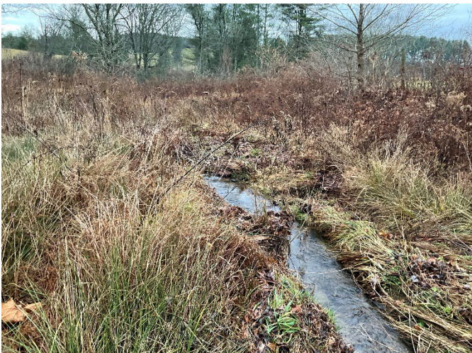
UT2A STA 431+25 – Phase I right bank repair area, looking downstream (12/7/2022)
