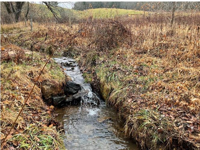
UT2 Reach 1 (Lower) STA 327+00 – Phase III rock cross vane added, looking upstream (12/7/2022)
