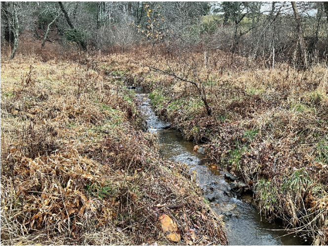
UT2 Reach 1 (Lower) STA 326+00 – 326+50 – Phase III buried channel rebuilt, rock cross vanes and riffles added, looking upstream (12/7/2022)
