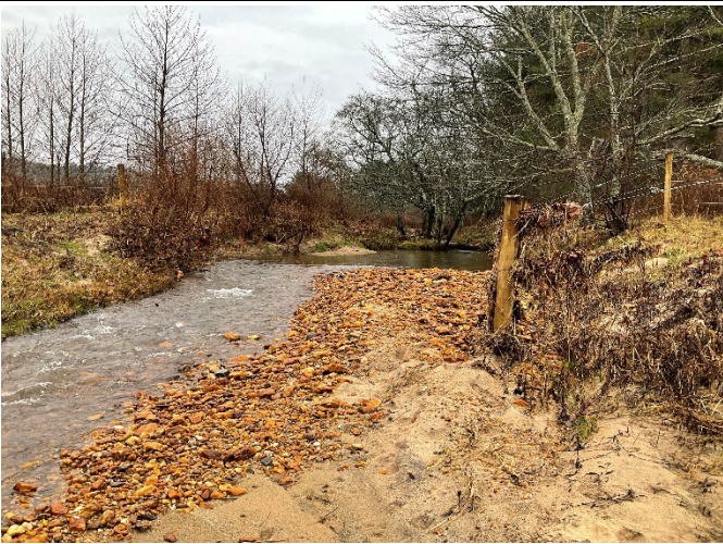
LPC Reach 2b STA 132+00 – Phase III ford crossing bar removal (still present), looking upstream (12/7/2022)
