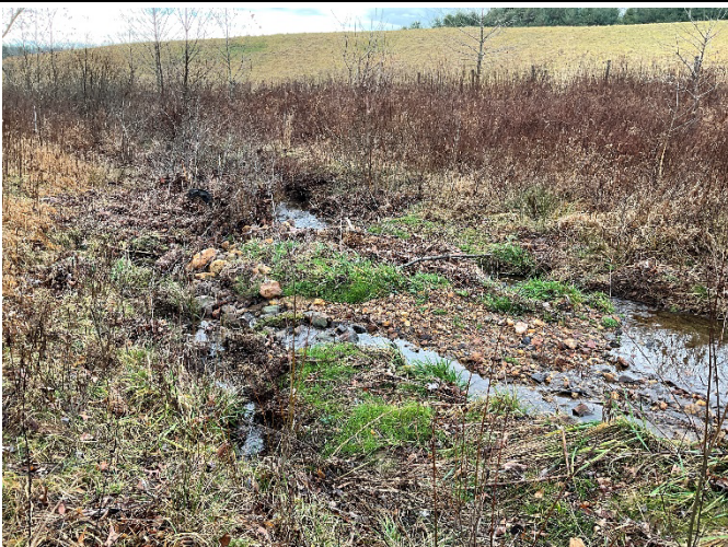
UT2 Reach 2 STA 333+50 – Mid channel sediment bar, looking downstream (12/7/2022)
