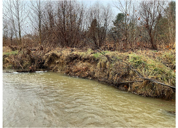
LPC Reach 1 STA 108+00 – Right bank scour, looking downstream (12/7/2022)
