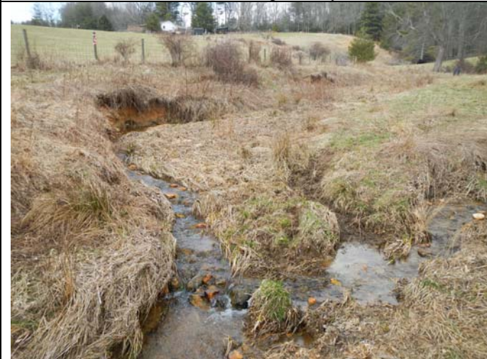
UT2, Reach 3 – bank erosion and wetland seep
