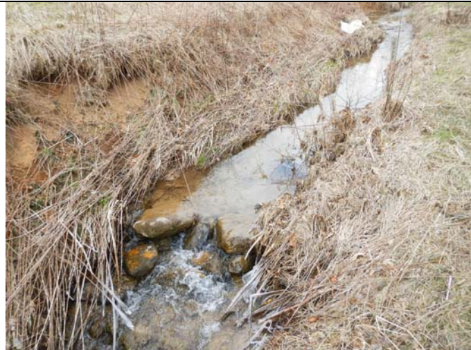
UT2, Reach 3 - headcut
