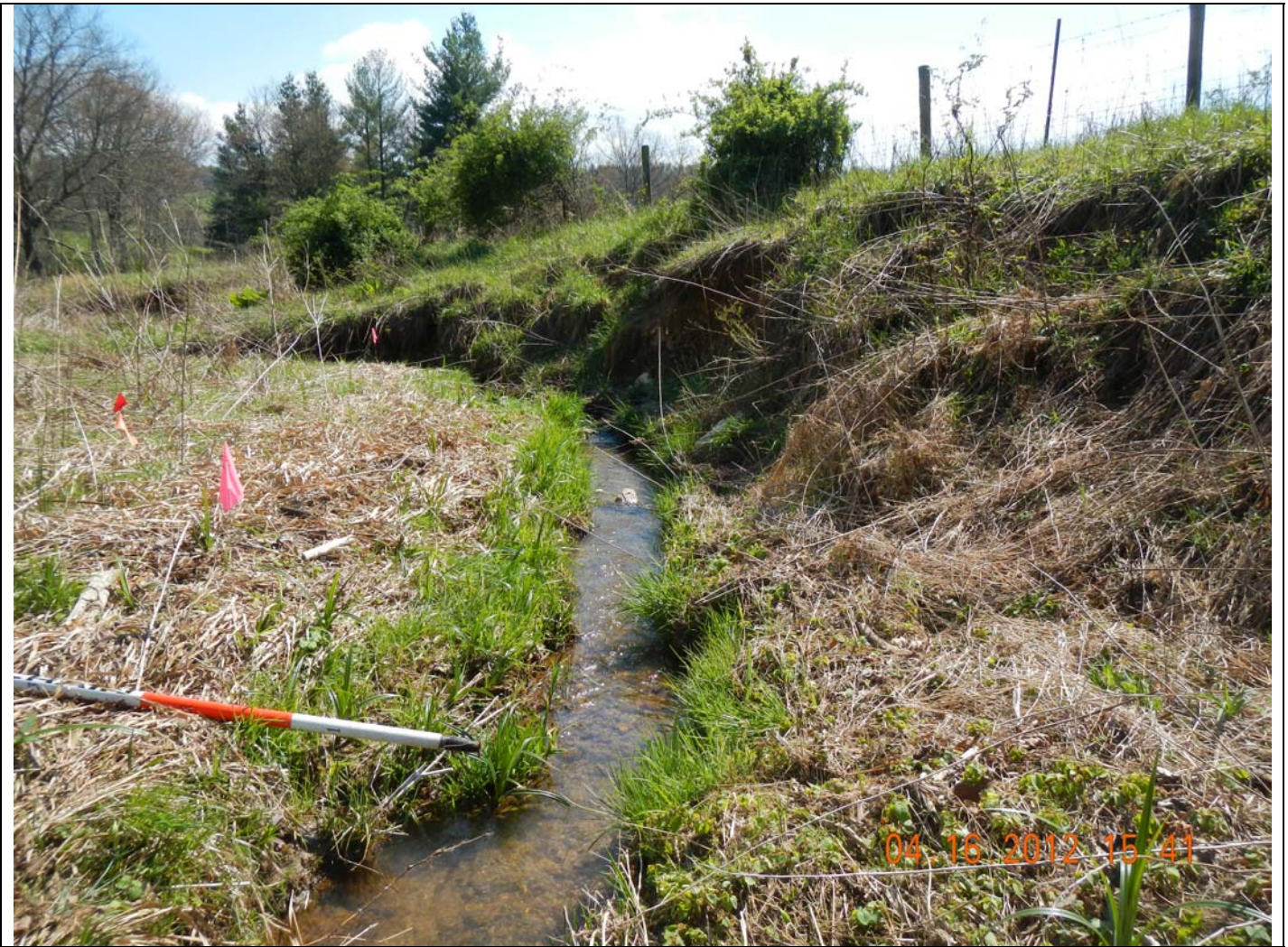
UT2A- XS7, looking downstream
