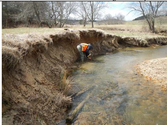
Little Pine, Reach 1 – reinstallation of bank pins on left bank
