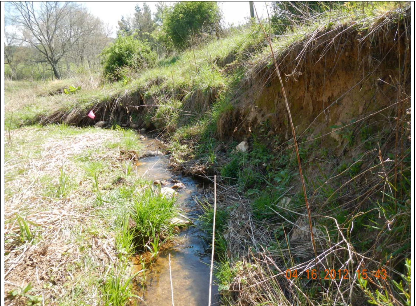
UT2A- XS8, looking downstream
