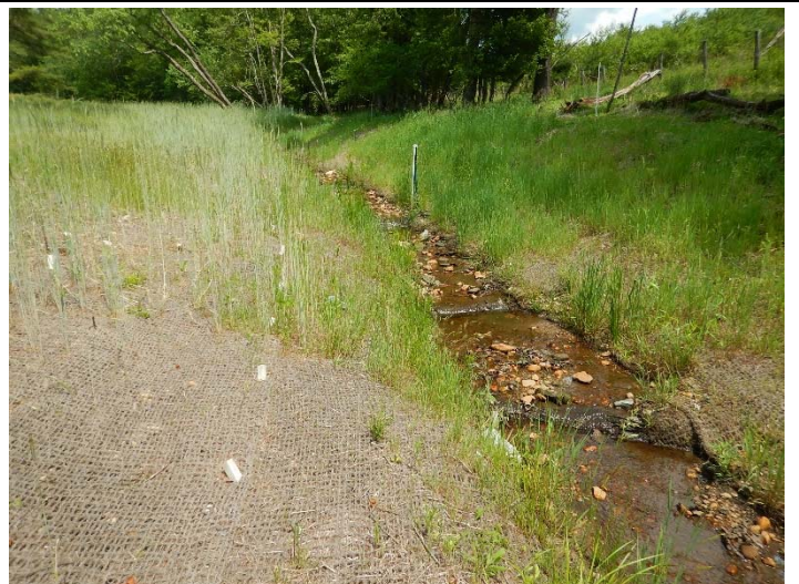
Photo Point 33 – looking upstream UT2b (05/31/2016)
