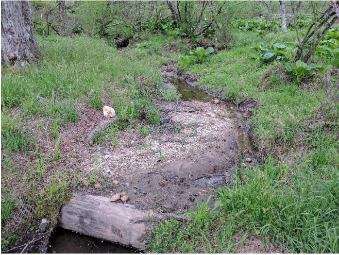
Photo Point 31 – UT2b, looking upstream (5/09/2017)
