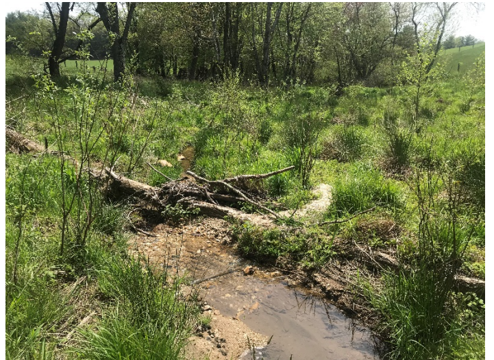
Photo Point 42 – UT2 Reach 1, looking downstream (04/30/2019)
