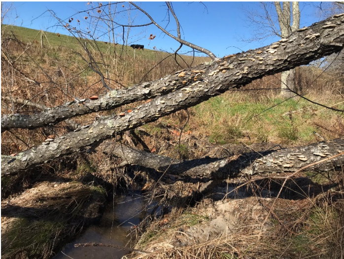
Photo Point 42 – UT2 Reach 1, looking upstream (12/08/2020)
