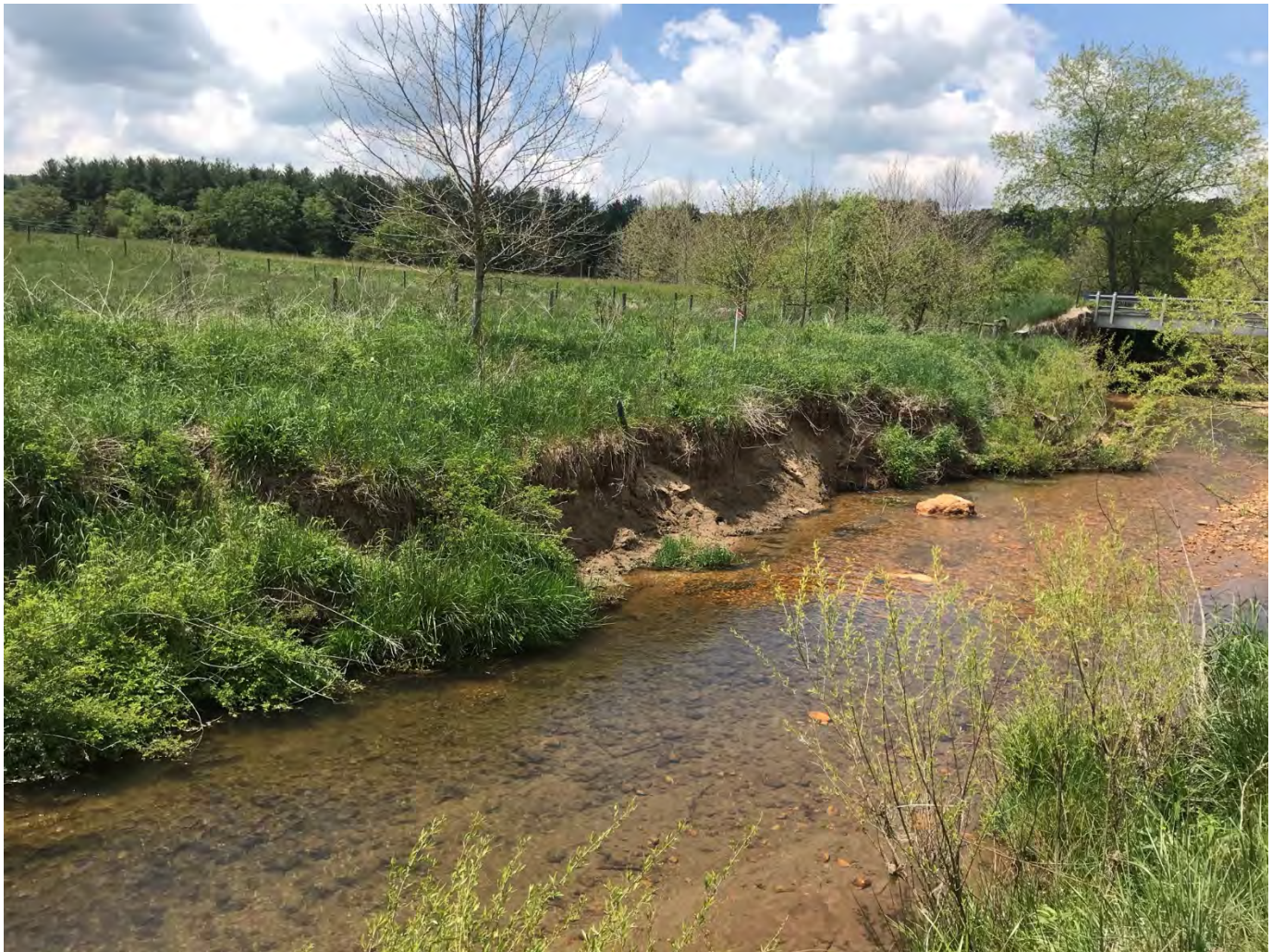
Little Pine Creek Repair Area: Bank erosion near station 131+00 (Location #13)
