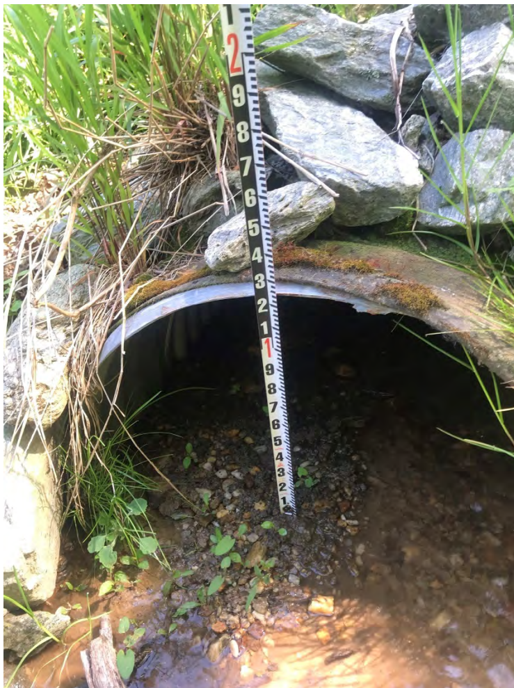
Culvert at Location #3
