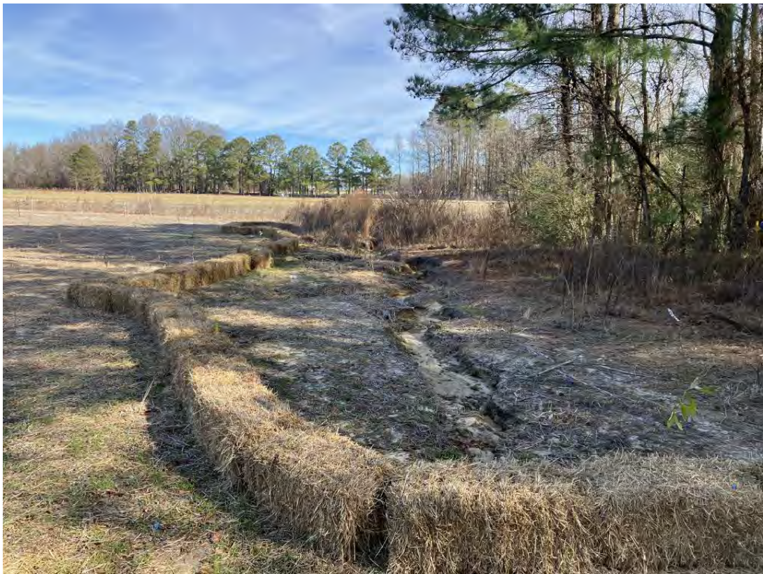
UT1 Erosion Reduction via Overland Flow Diversion (1/16/2023)
