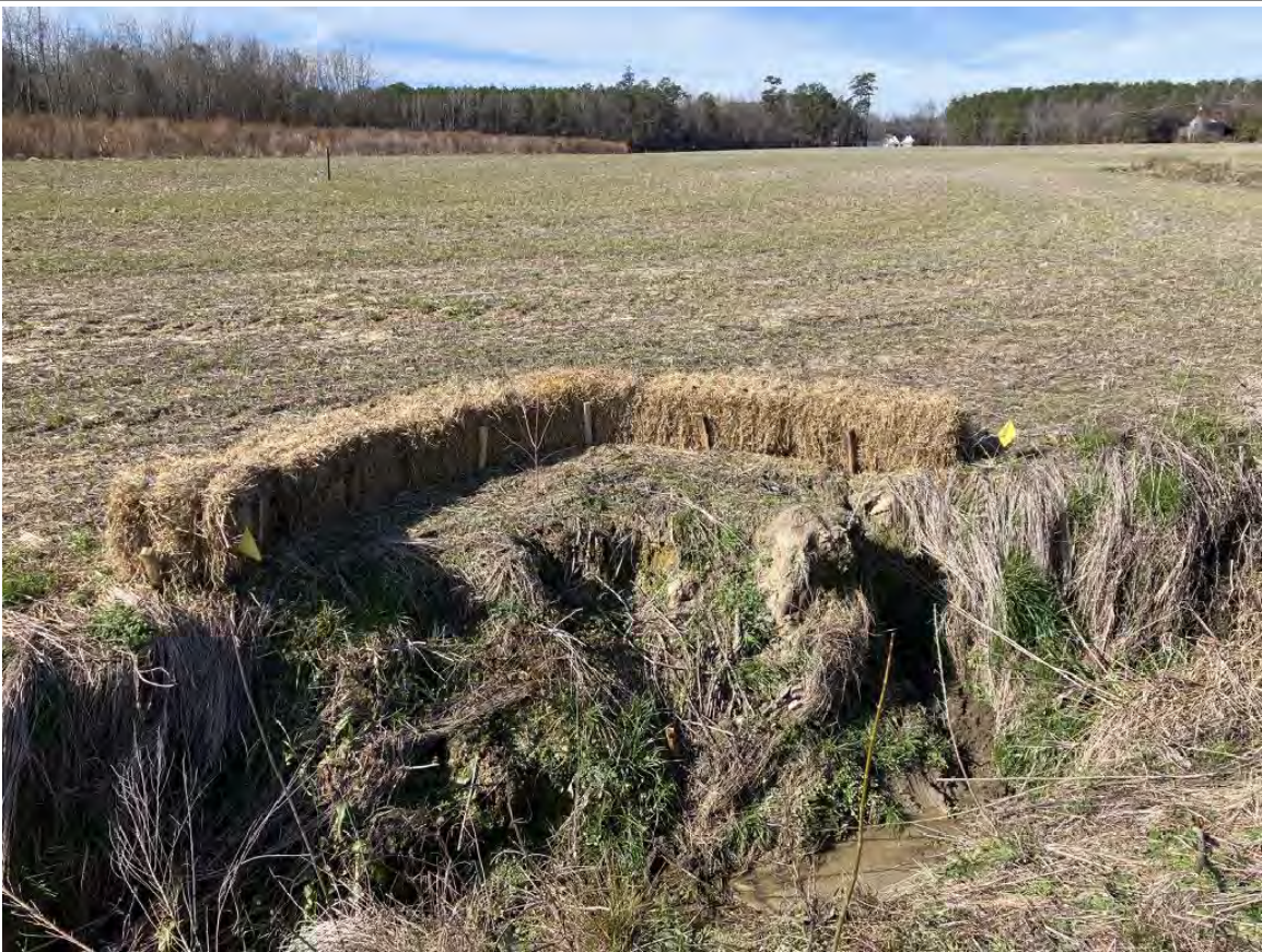
UT1 Erosion Reduction via Overland Flow Diversion and Live Stakes (1/16/2023)
