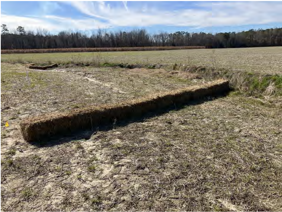
UT1 Erosion Reduction via Overland Flow Diversion (1/16/2023)
