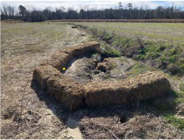
UT1 Erosion Reduction via Overland Flow Diversion and Live Stakes (1/16/2023)
