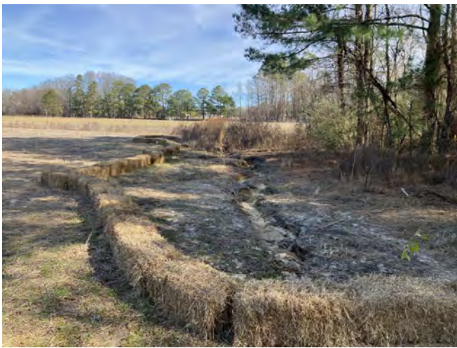
UT1 Erosion Reduction via Overland Flow Diversion (1/16/2023)
