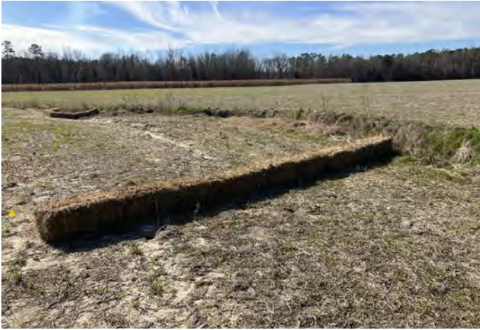
UT1 Erosion Reduction via Overland Flow Diversion (1/16/2023)
