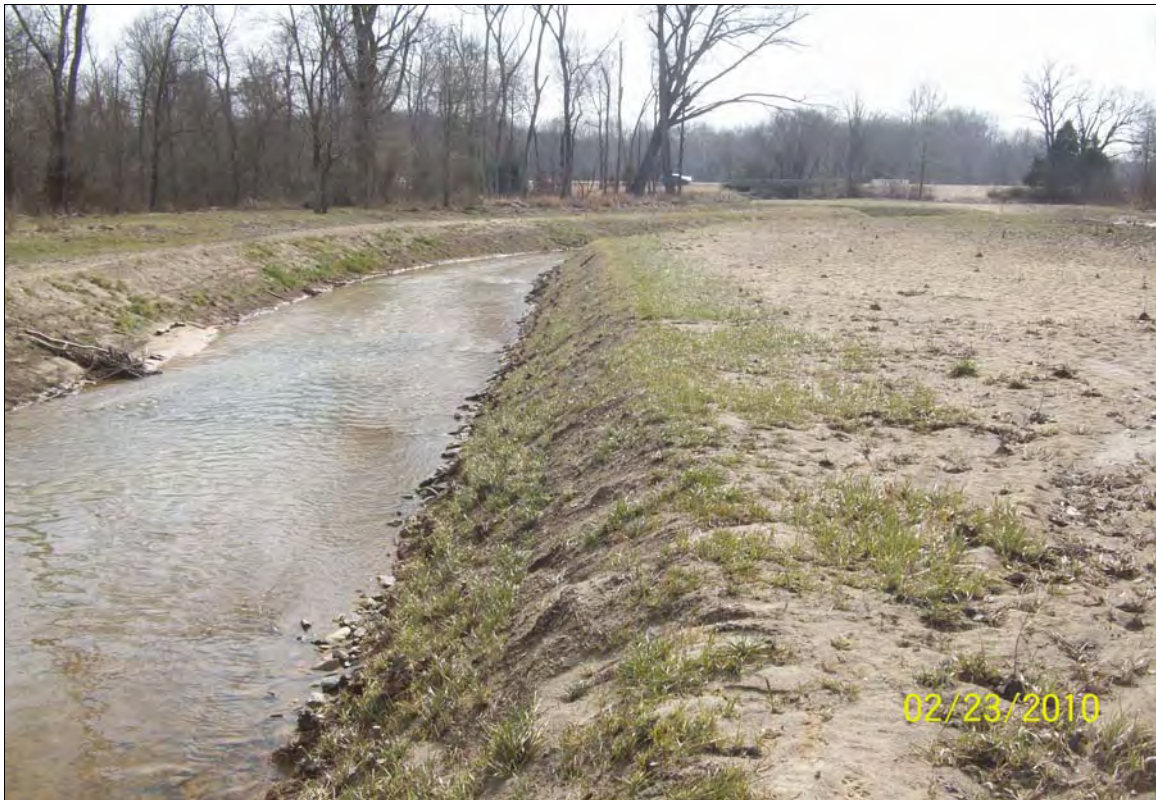
Photo Point 2d: View looking downstream taken near Station 17+40. 2/23/10 – Baseline
