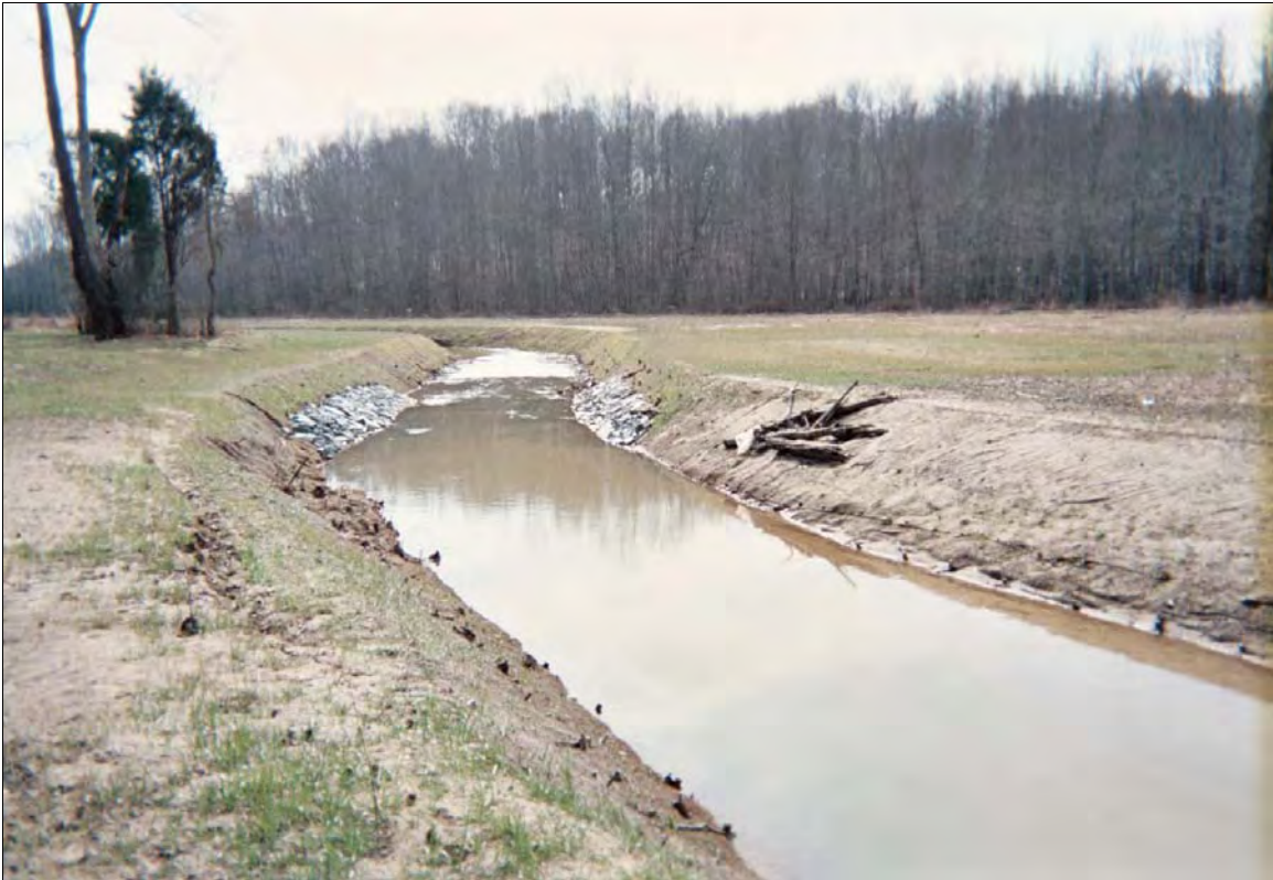
Photo Point 1d: View looking downstream near Station 11+10. 2/23/10 – Baseline
