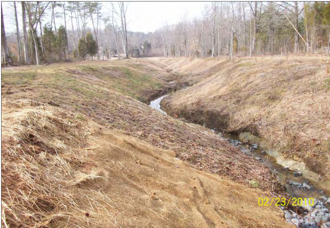
Photo Point 5: View looking downstream near Station 50+00. 2/23/10 – Baseline
