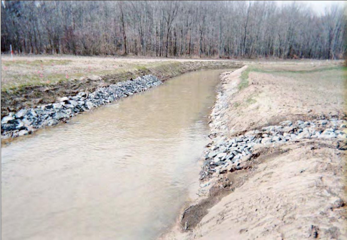
Photo Point 3u: View looking upstream near Station 22+25. 2/23/10 – Baseline
