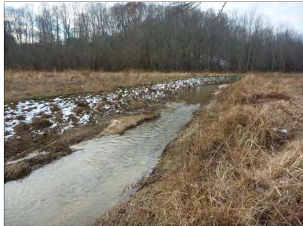
Photo Point 3u: View looking upstream near Station 22+25. 12/10/10 – MY-01
