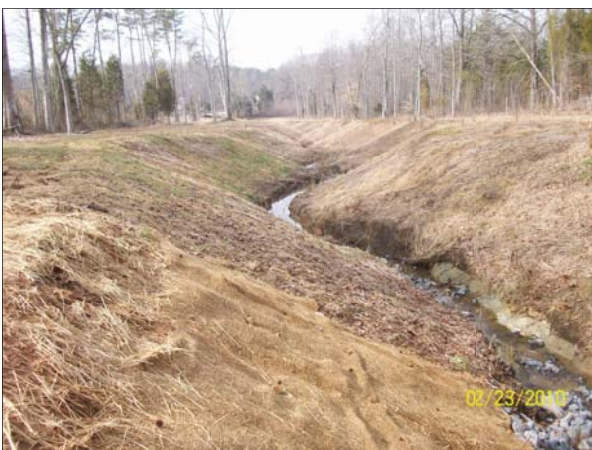
Photo Point 5: View looking downstream near Station 50+00. 2/23/10 – Baseline
