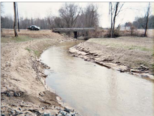
Photo Point 3d: View looking downstream near Station 22+25. 2/23/10 – Baseline
