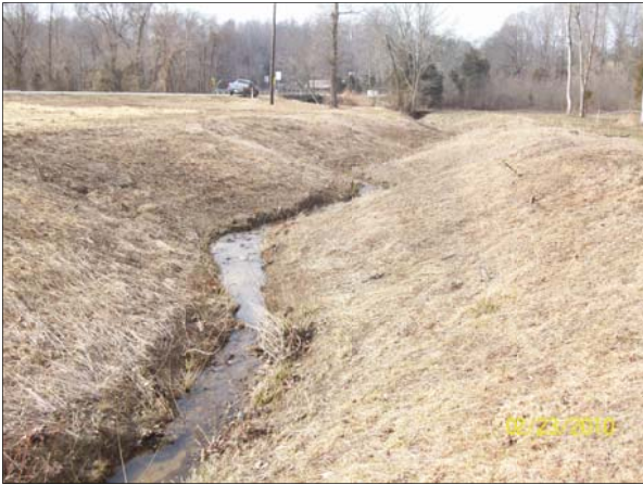
Photo Point 6d: View looking downstream near Station 54+90. 2/23/10 – Baseline
