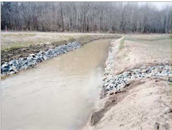
Photo Point 3u: View looking upstream near Station 22+25. 2/23/10 – Baseline
