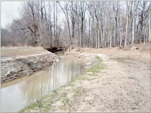
Photo Point 1u: View looking upstream near Station 11+10. 2/23/10 – Baseline
