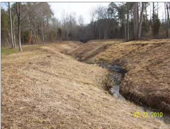
Photo Point 6u: View looking upstream near Station 54+90. 2/23/10 – Baseline
