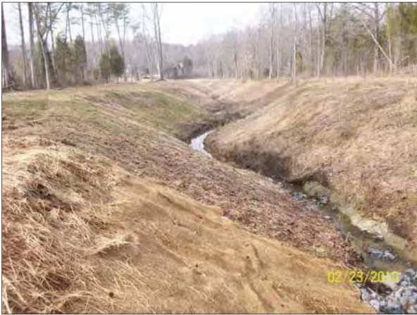
Photo Point 5: View looking downstream near Station 50+00. 2/23/10 – Baseline
