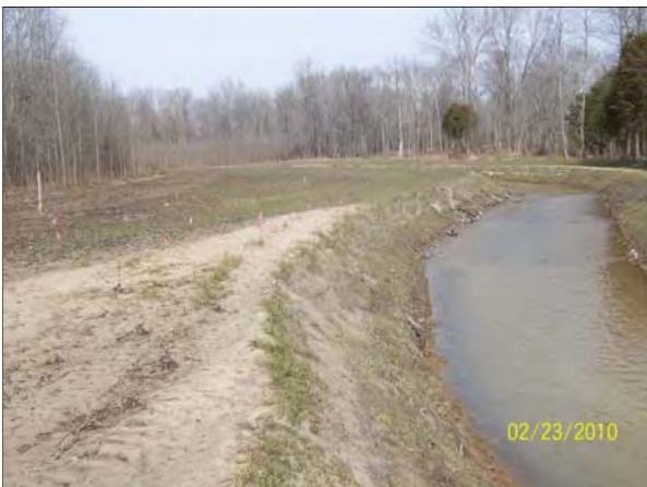
Photo Point 2u: View looking upstream taken near Station 17+40. 2/23/10 – Baseline
