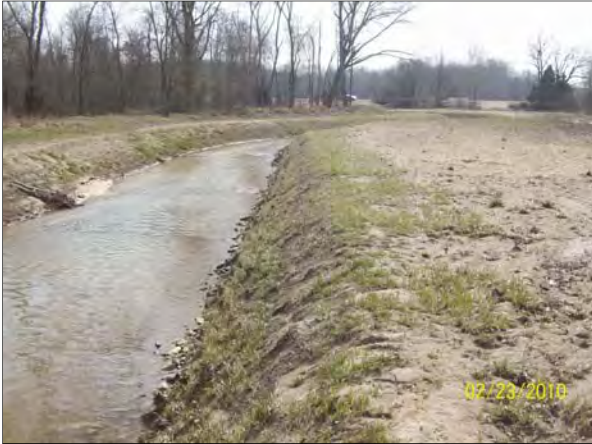
Photo Point 2d: View looking downstream taken near Station 17+40. 2/23/10 – Baseline
