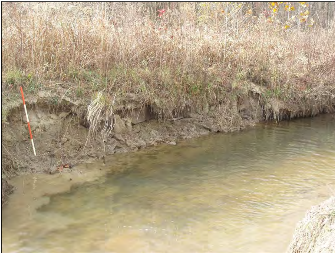
11/21/2013 MY04 – bank erosion (Stationing 20+50)
