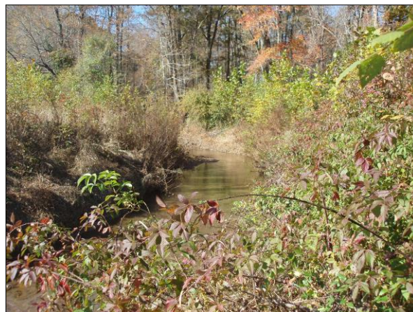
Photo Point 1u: View looking upstream near Station 11+10. 11/10/2014 – MY-05
