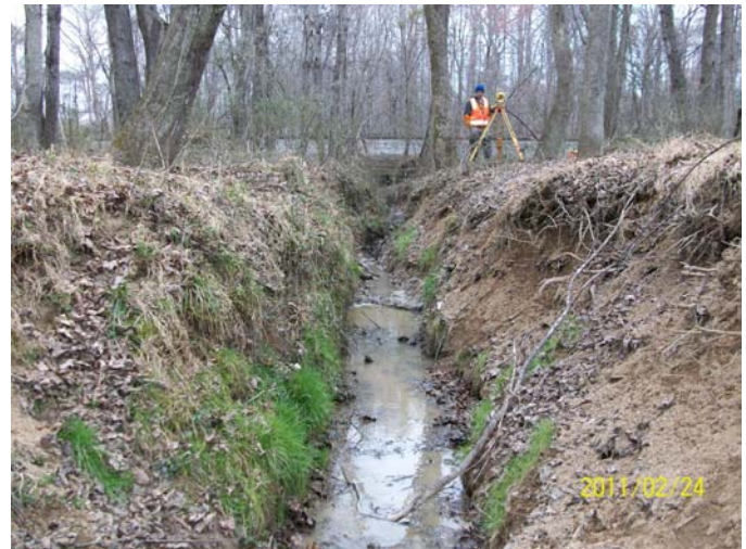
UT1, facing upstream to culvert crossing – Stream Mitigation Site
