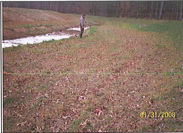
As-built Survey: January 2008
