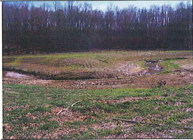
As-built Survey: January 2008
