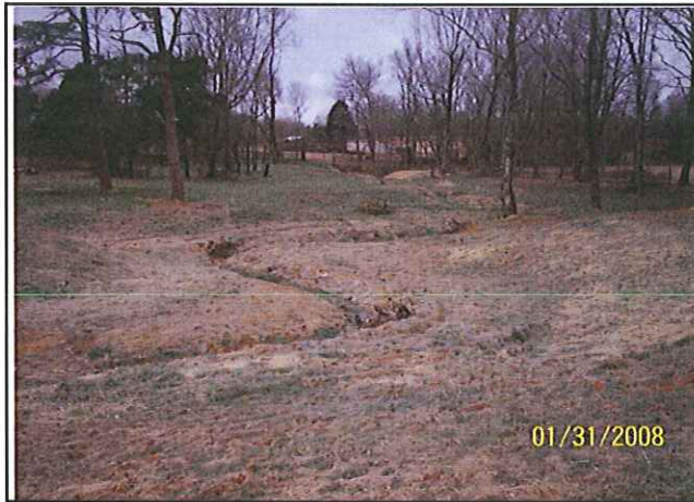
As-built Survey: January 2008
