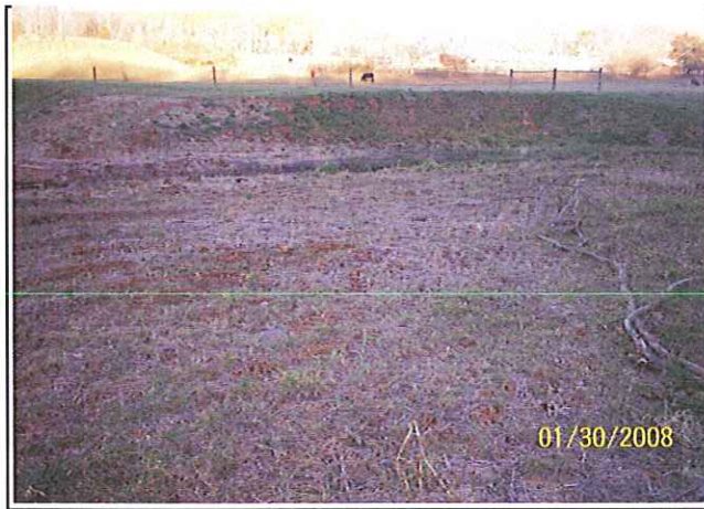
As-built Survey: January 2008
