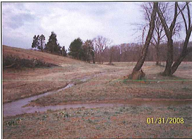
As-built Survey: January 2008
