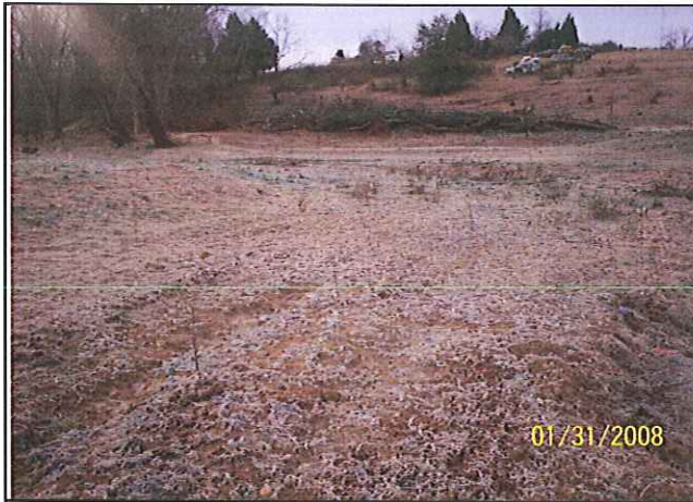
As-built Survey: January 2008
