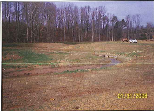
As-built Survey: January 2008
