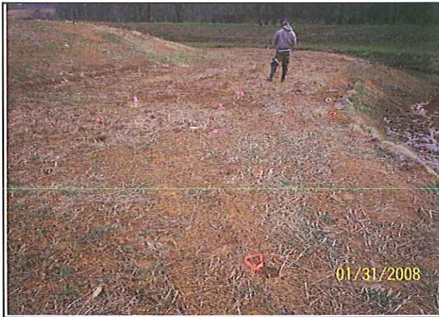
As-built Survey: January 2008
