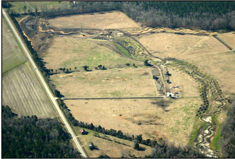
Main channel looking toward the top of the Site
