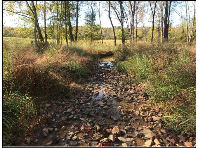
PP-8: Reach 1, view downstream, Station 23+00
