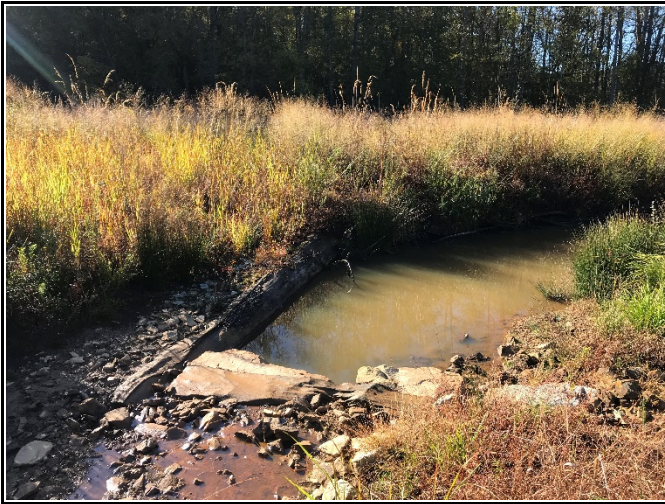
PP-3: Reach 1, view downstream, Station 13+75
