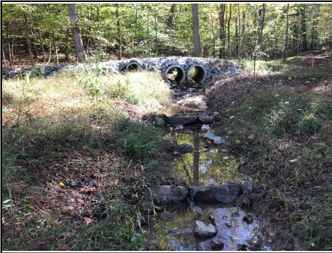
PP-23: Reach 3, view upstream, Station 10+50
