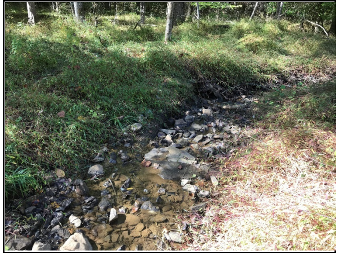
PP-26: Reach 3, view downstream, Station 12+75
