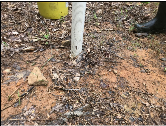
Debris jam by manual crest gauge on upper R3 (photo: 6/19/19)
