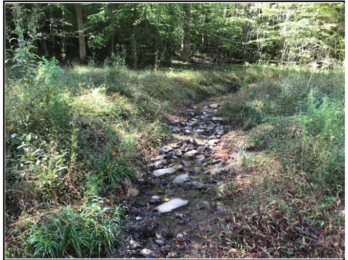
PP-24: Reach 3, view downstream, Station 10+75
