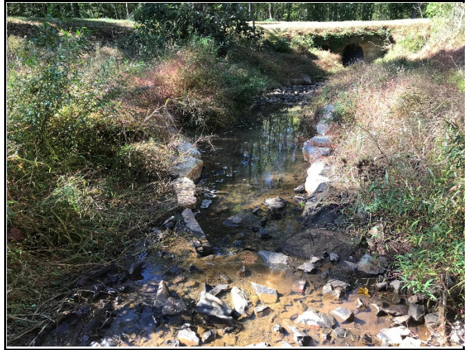
PP-20: Reach 1, view downstream, Station 41+00
