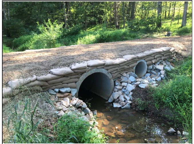
Repaired pipe crossing on R3 (downstream side) at Station 16+50
