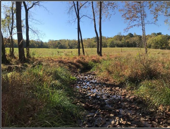
PP-9: Reach 1, view downstream, Station 25+00
