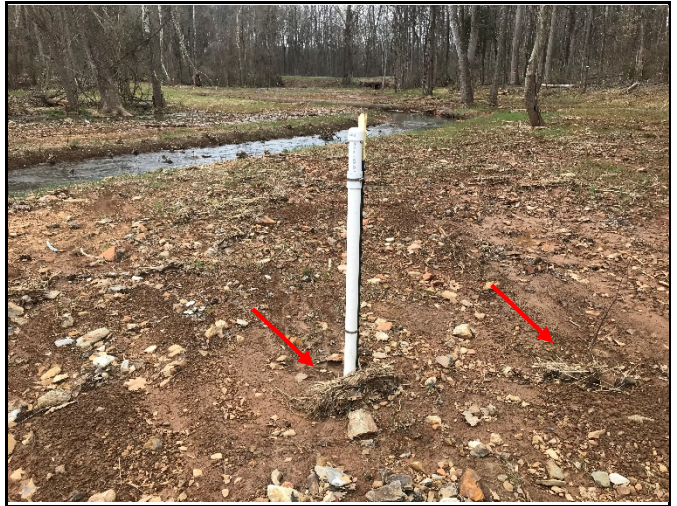
Debris jams by automated crest gauge and tree stem on lower R1 floodplain (photo: 3/7/19)
