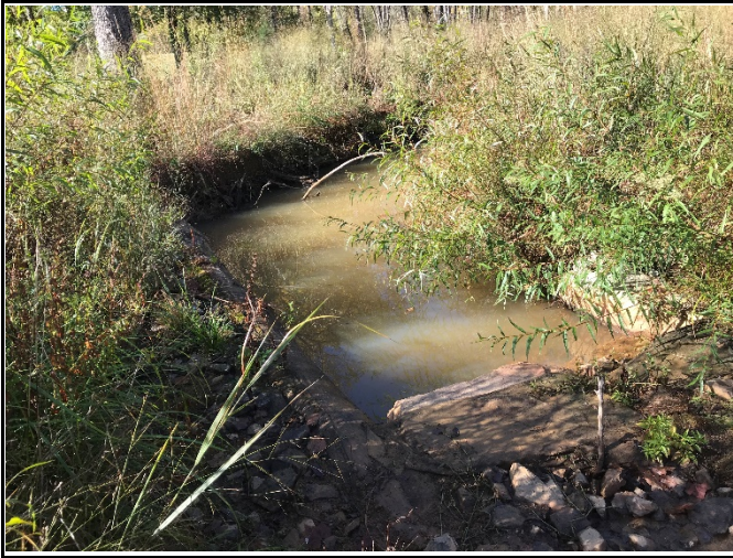
PP-7: Reach 1, view downstream, Station 21+50
