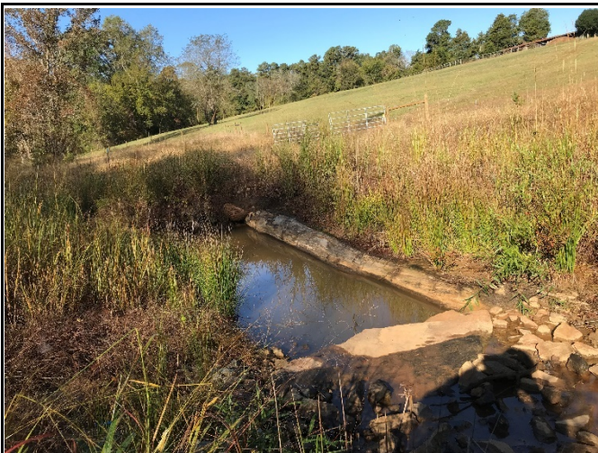
PP-5: Reach 1, view downstream, Station 16+50
