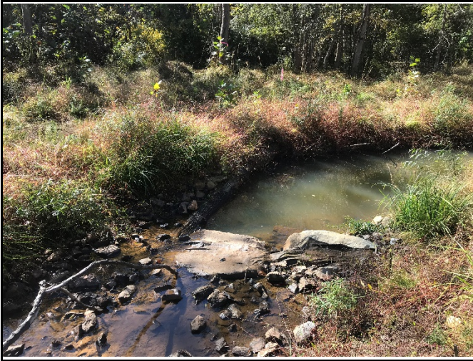
PP-19: Reach 1, view downstream, Station 39+75
