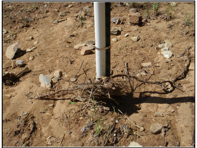
Debris jam by manual crest gauge on upper R1 (photo: 4/18/19)
