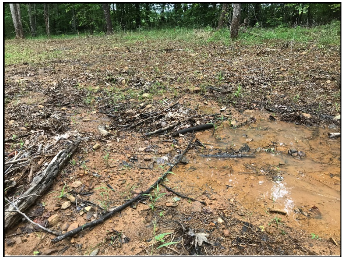
Scour flow paths and debris in floodplain of upper R3 (photo: 6/19/19)
