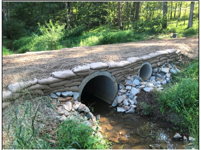
Repaired pipe crossing on R3 (downstream side) at Station 16+50 in Sept. 2019
