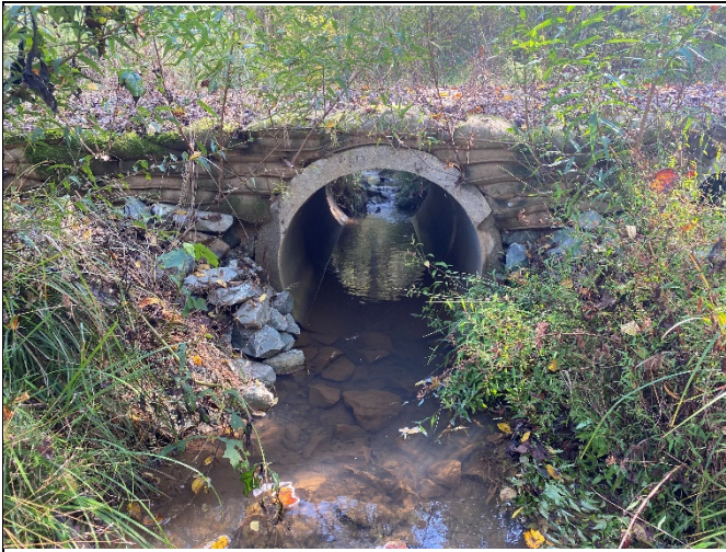
Pipe at crossing on R3 at Station ~16+30 (10/13/20)
