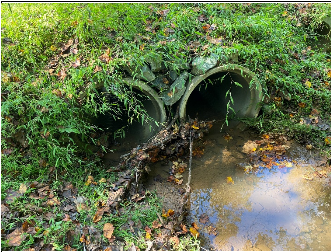
Pipes at crossing at top of R3 at Station 10+00 (10/13/20)
