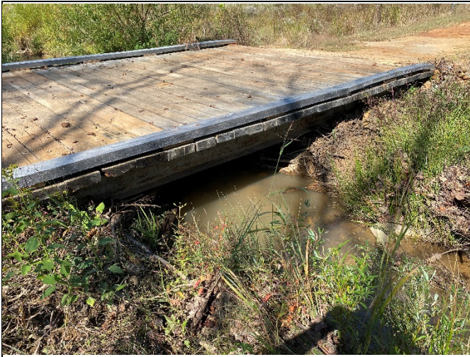
Bridge on R1 at Station ~18+20 (10/13/20)
