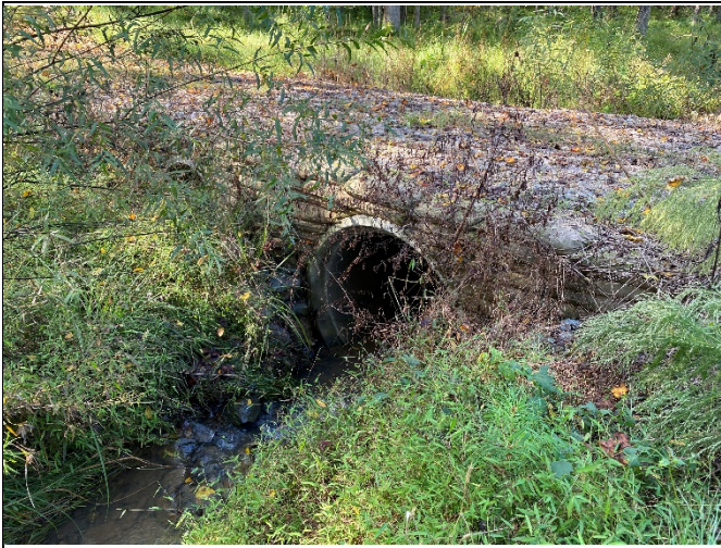
Repaired pipe crossing on R3 (upstream side) at Station 16+20 in October 2020
