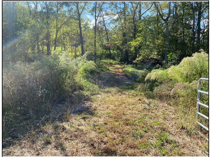
Crossing over pipe on R3 at Station ~16+30 (10/13/20)
