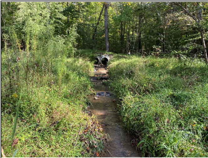
PP-23: Reach 3, view upstream, Station 10+50
