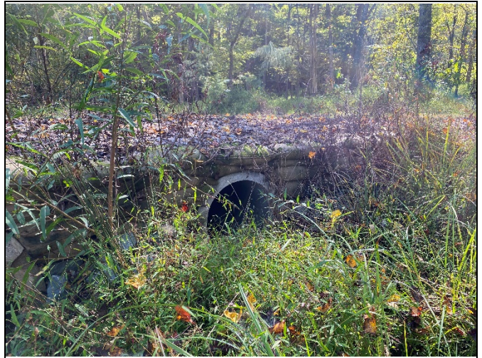
Repaired pipe crossing on R3 (downstream side) at Station 16+50 in October 2020
