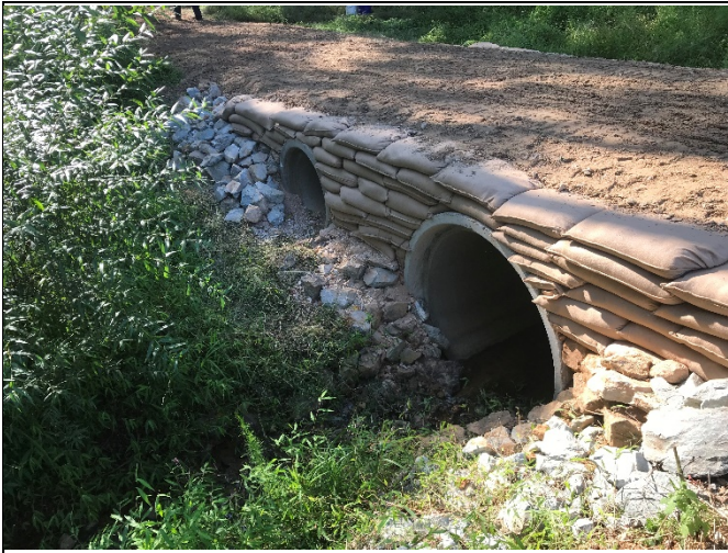
Repaired pipe crossing on R3 (upstream side) at Station 16+20 in Sept. 2019
