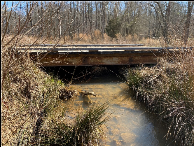
Bridge on R1 at Station ~18+20 (3/11/21)
