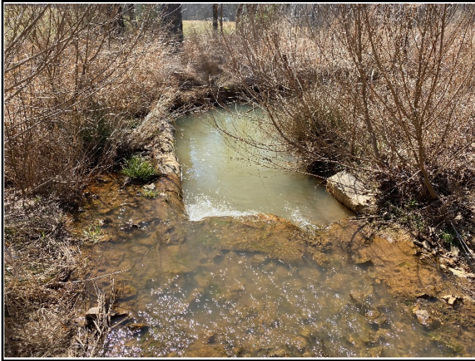
PP-7: Reach 1, view downstream, Station 21+50
