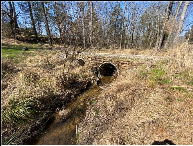
Pipe crossing on R3 at Station ~16+30 (3/11/21)
