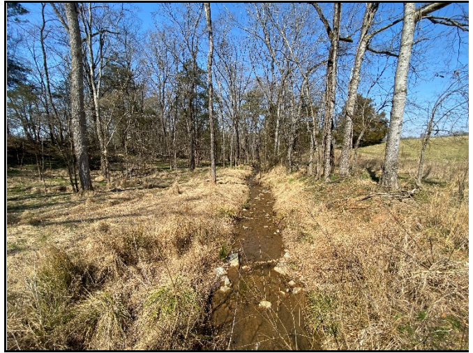
PP-28: Reach 3, view downstream, Station 16+25
