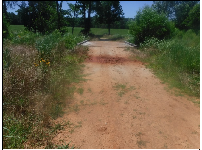
Stable crossing over bridge on R1 at Station ~18+20 (6/21/21)
