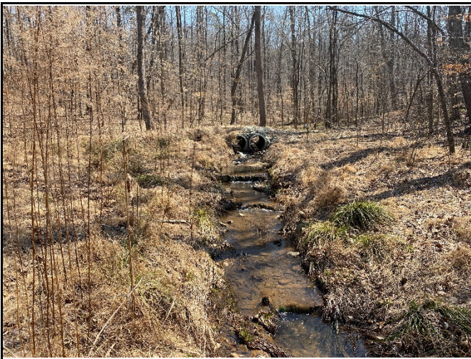
PP-23: Reach 3, view upstream, Station 10+50
