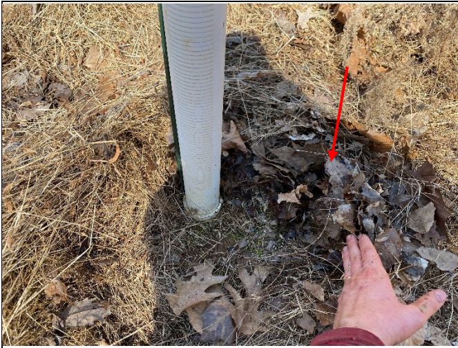
Debris jammed up against crest gauge base (pushed back for photo) on upper R3 (photo from 3/11/21)
