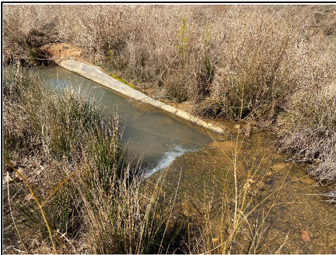
PP-5: Reach 1, view downstream, Station 16+50
