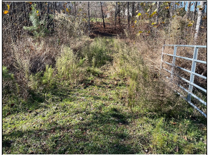
Stable pipe crossing on R3 at Station ~16+30 (11/21/22)
