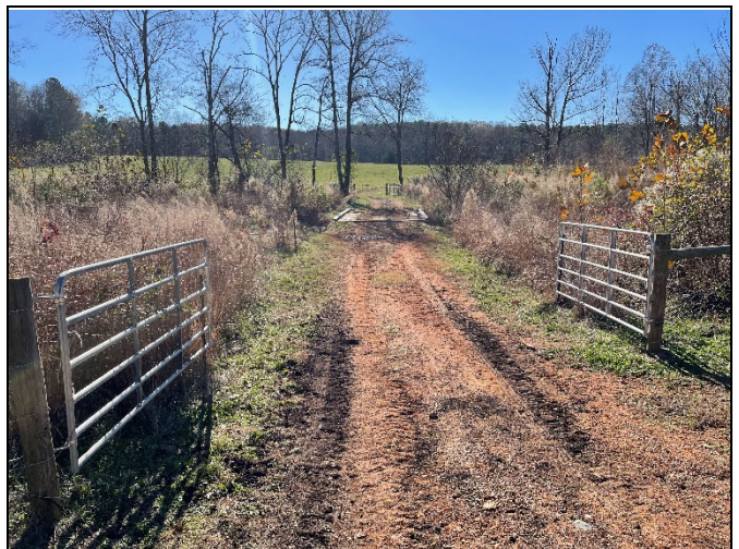
Stable bridge crossing over Reach 1 (11/21/22)
