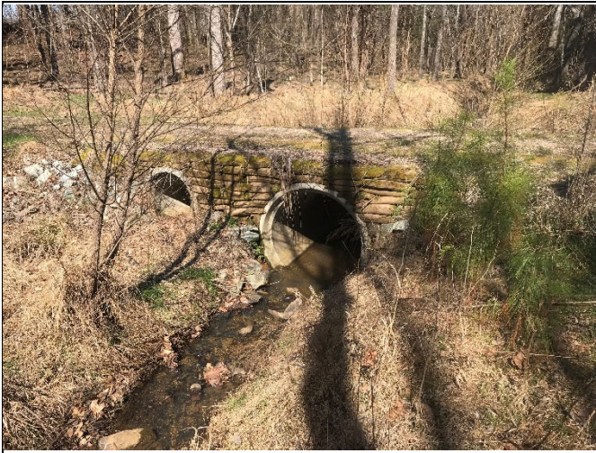
Pipe crossing on R3 at Station ~16+30 (3/15/22)
