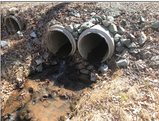
Pipes at crossing at top of R3 at Station 10+00 (3/15/22)
