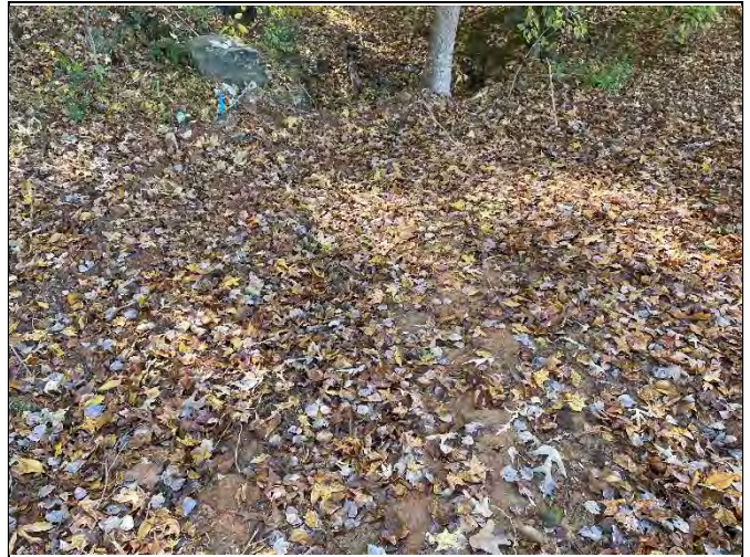
Encroachment area filled back in and graded out (photo from (11/1/23))
