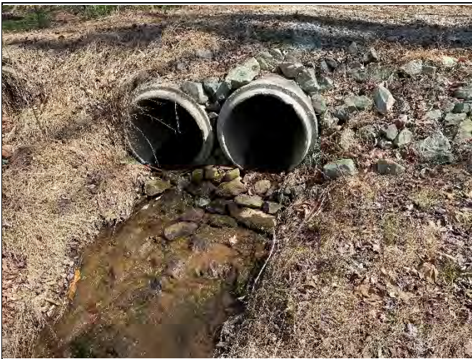
Pipes at crossing at top of R3 at Station 10+00 (3/23/23)
