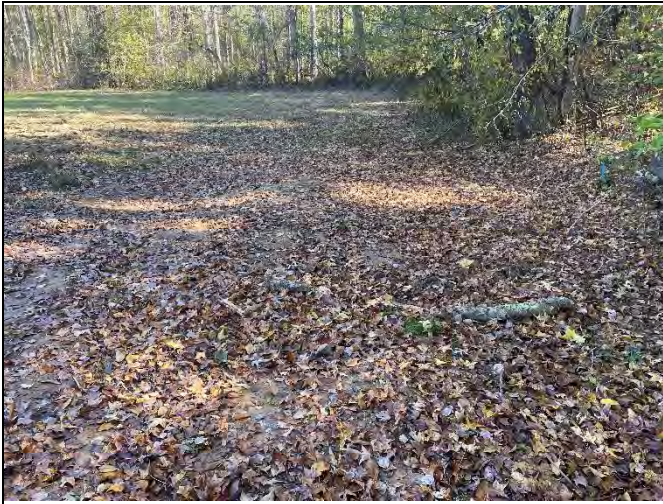
Encroachment area filled back in and graded out (photo from (11/1/23))
