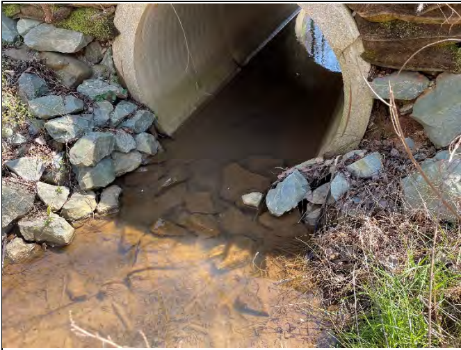
Pipe crossing on R3 at Station ~16+30 (3/23/23)
