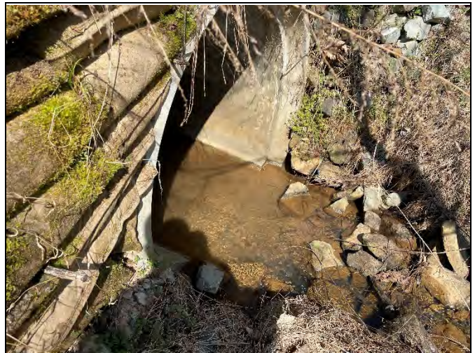
Pipe crossing on R3 at Station ~16+30 (3/23/23)
