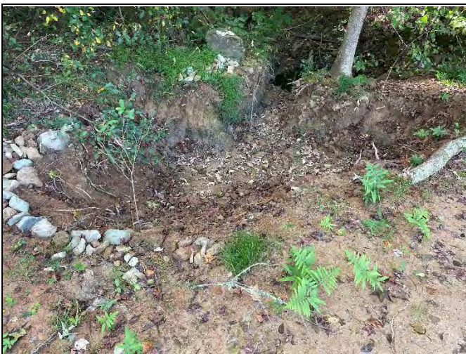
Encroachment area at the head of R2 (8/5/2023)
