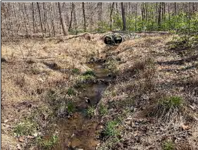
PP-23: Reach 3, view upstream, Station 10+50
