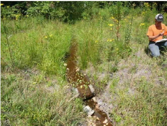
Photo 56. UT2, Photo Point 28 – Station 1+10 (August 2015) upstream view from right bank and confluence.
