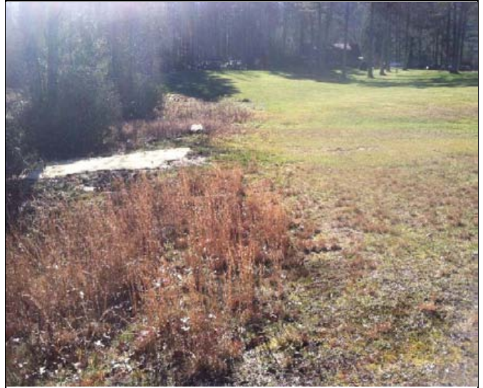
Photo 9. View along the easement line after the pipe was removed. Perspective is similar to Photo 5 but from the opposite direction.
