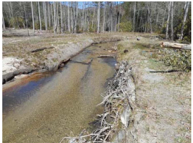
Photo 47. Logan Creek Photo Point 23 – Station 7+70 (March 2016) upstream view from left bank.
