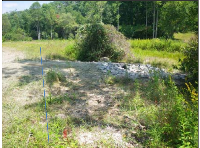
Photo 5. Encroachment by landowner who installed a drainpipe to have its outfall within the easement.
