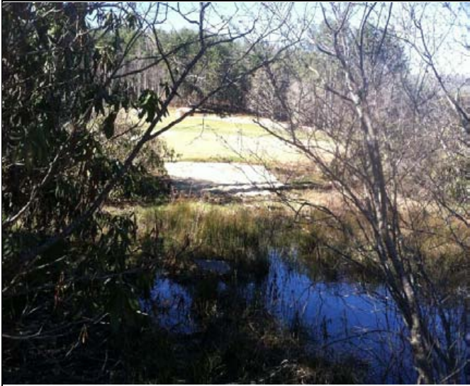
Photo 8. Perspective similar to that of Photo 6 showing the area after the pipe was removed.
