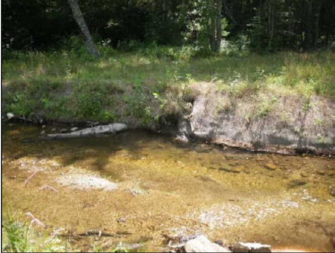
Photo 1. Bank Scour – Station 2+80, Small area of bank scour due to soft place in bank eroding on high flow.
