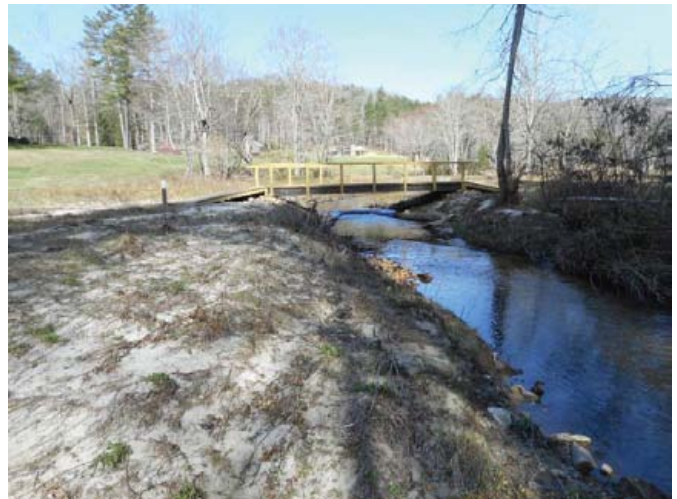
Photo 16. Logan Creek Photo Point 8b – Station 29+25 (March 2016) upstream view from right bank.
