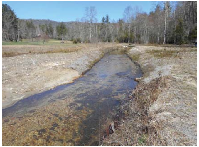
Photo 22. Logan Creek Photo Point 11 – Station 23+20 (March 2016) upstream view from left bank.
