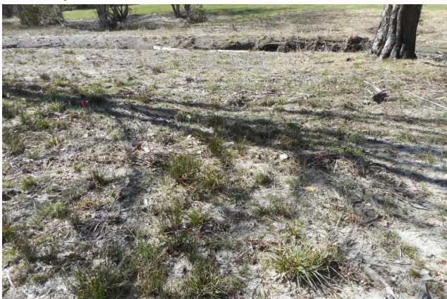
Wreck lines well back from the stream, indicating wide flooding of the floodplain during storms of late December 2015 and early February 2016.
