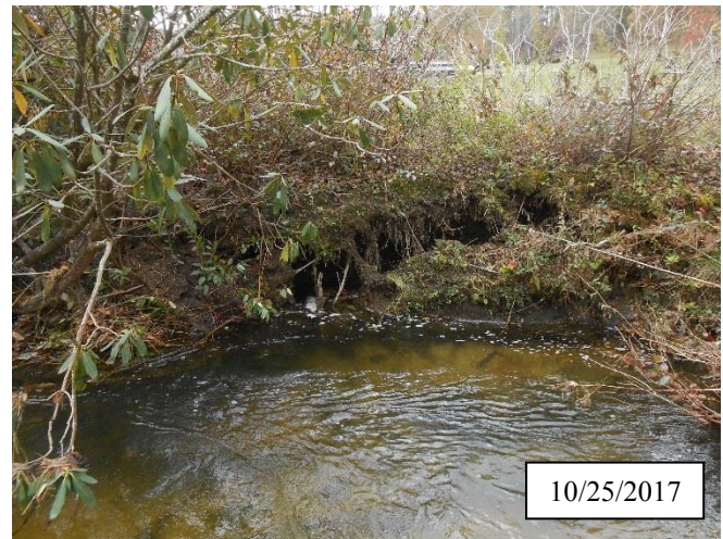
Photo 16. CPA 3-4 – Station 11+50, small bank slump (approx. 8 ft.) along right bank of main stem. Will be monitored to see if the bank stabilizes in MY4
