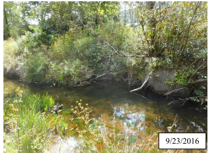
Photo 8. CPA 2-4 – Station 11+70, scour area noted in MY2 has stabilized for the most part. Livestakes were planted in the scour area as well as the bank downstream of the problem area in October 2017.
