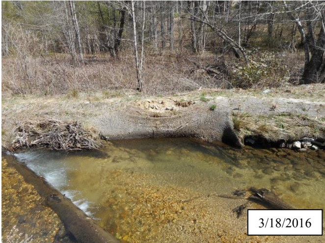
Photo 1. CPA 2-1 – Station 2+10, small area of bank scour caused by flooding of December and January.
