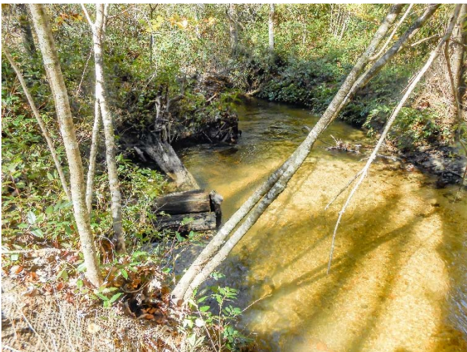
Photo 11. Logan Creek Photo Point 6 – Station 32+70 (October 2017) downstream view from left bank.
