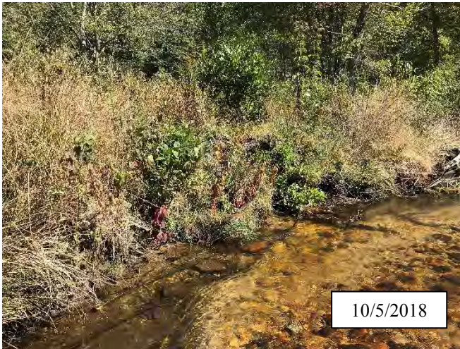
Photo 15. CPA 2-5 – Station 26+60, Scour area has revegetated and stabilized.
