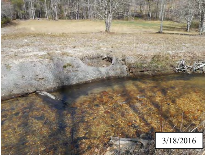
Photo 13. CPA 2-5 – Station 26+60, small area of bank scour caused by flooding of December and January 2016.
