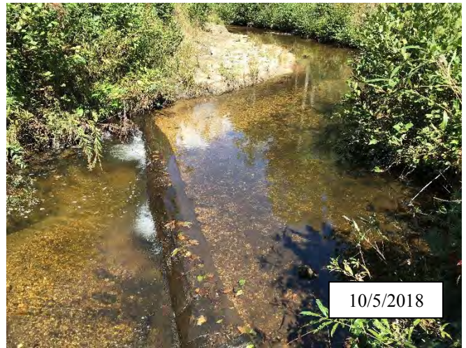
Photo 20. CPA 3-1 – Log structure has stabilized and is no longer piping.
