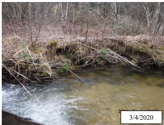
Photo 4. CPA 2-1, Scour area is stable and supporting vegetation, late winter photo (3-2020).
