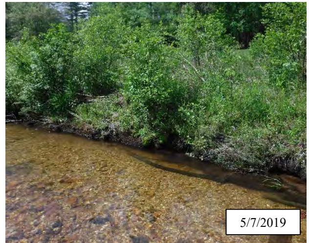
Photo 24. CPA 2-6 – Station 27+00, scour area remained vegetated and stable in 2019.
