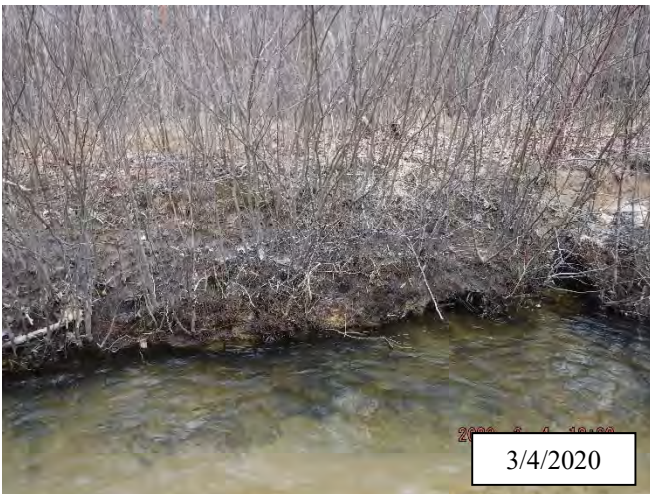
Photo 31. CPA 3-2 – Area has stabilized and is fully vegetated, in late winter 2020.
