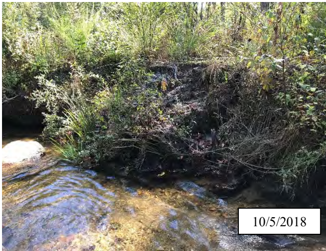
Photo 11. CPA 2-3 – Station 4+60, bank scour area has vegetated but not completely stable.
