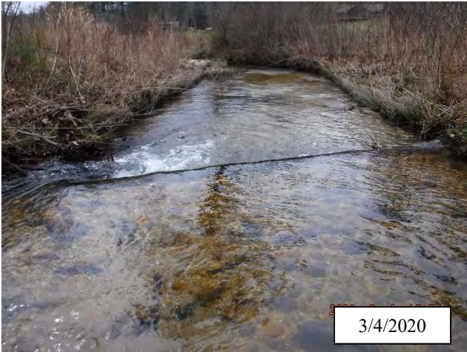
Photo 34. CPA 3-3 – Station 14+75, Log structure continues to be stable in late winter 2020.
