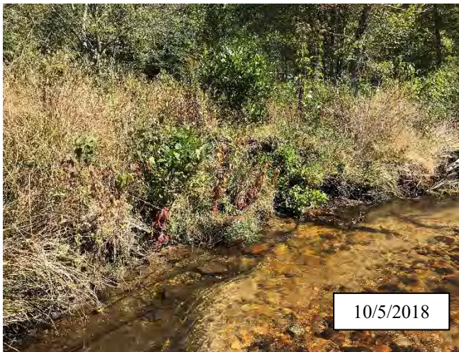
Photo 19. CPA 2-5 – Station 26+60, Scour area has revegetated and stabilized.
