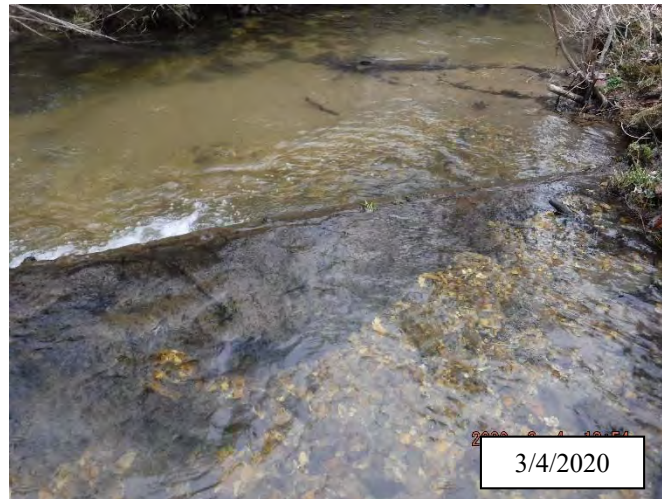
Photo 8. CPA 2-2 – Log structure has remained stable and not piping, late winter photo (3-2020) after multiple high water events.
