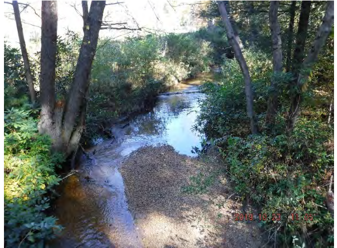
Photo 14. Logan Creek Photo Point 7 – Station 32+00 (October 23, 2019) upstream view from bridge.
