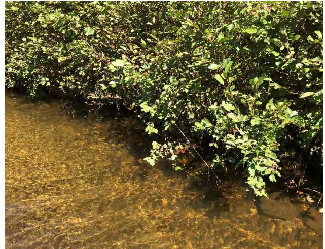
Photo 30. CPA 3-2 – Area has stabilized and is fully vegetated.
