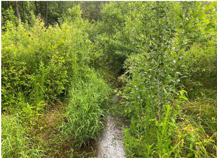
Photo Point 10 – UT1 Reach 2B, view upstream (07/08/2021)
