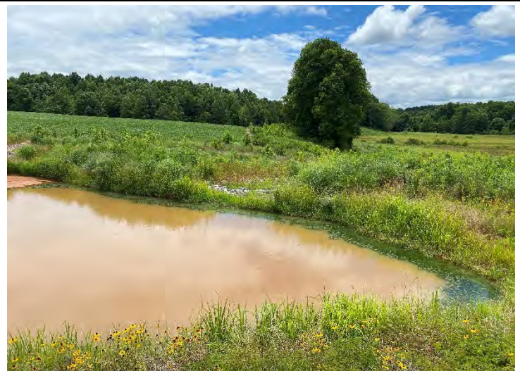
Photo Point 44 – BMP 4 above UT2B, outlet view (07/08/2021)
