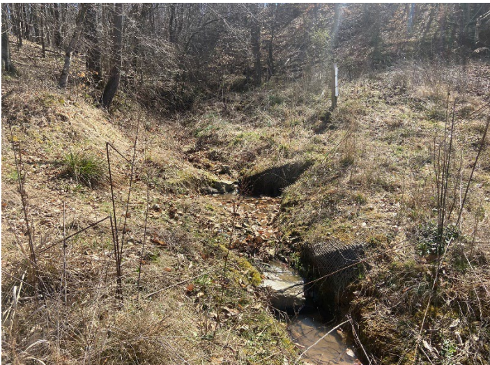
Photo Point 27 – UT2A, view upstream (03/14/2022)
