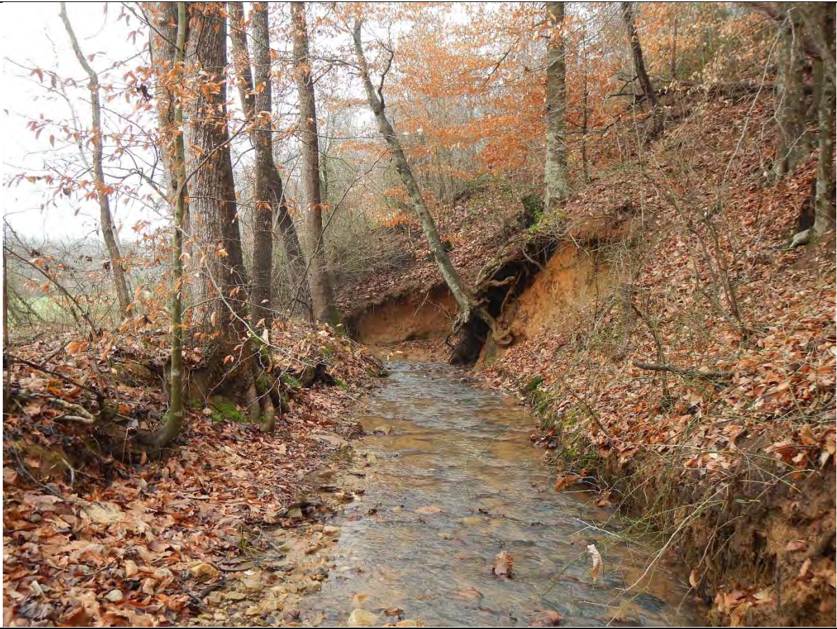
UT1 – Reach 2B, Consistent bank erosion, mass wasting of valley wall, and embedded riffle substrate.
