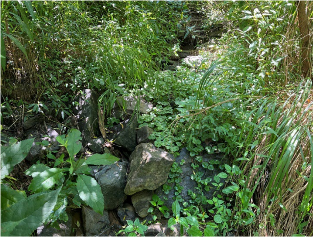
UT1 Reach 1, STA 107+10 – Structure piping (07/25/2023)
