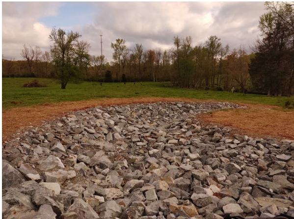
(3) PS2 (looking north towards restoration area)
