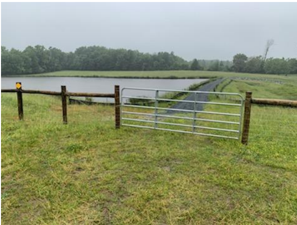
(6) PS4 (looking west towards dam)
