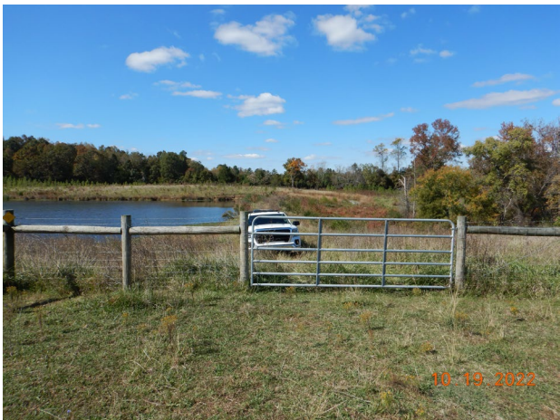
(6) PS4 (looking west towards dam)
