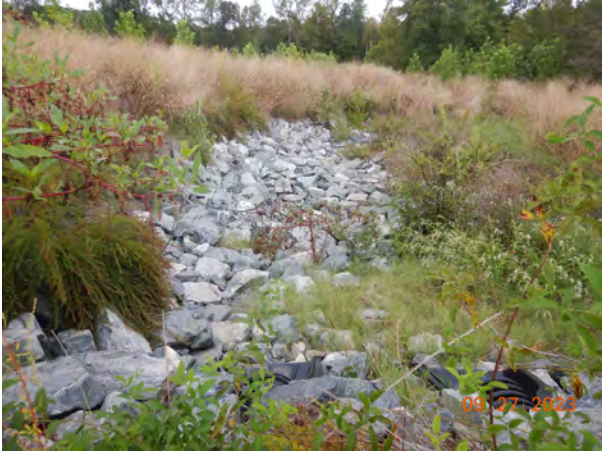
(2) PS2 (looking north towards restoration area)
