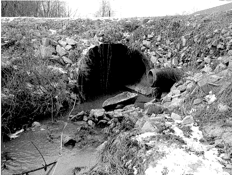
1. Beginning of project looking upstream at culvert under NC 39.
