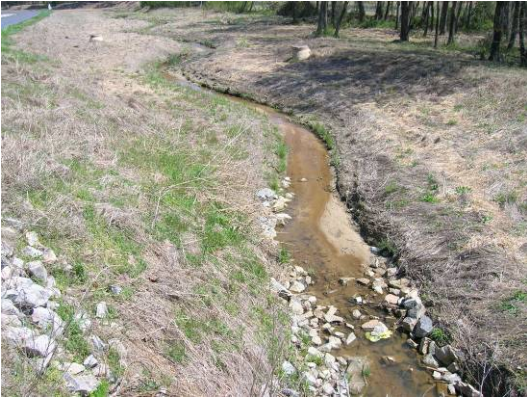
Photo Point 1. Downstream From Culvert at NC39 (from SREV 10+00)
