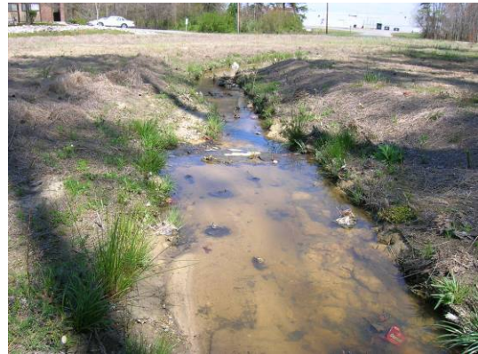
Photo Point 8. Downstream of Veg Plot #03 to Curve C-16
