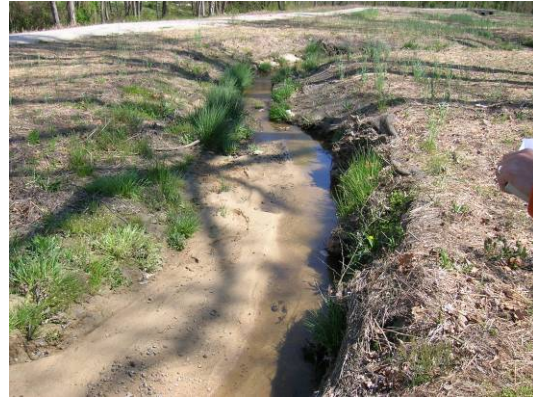
Photo Point 11. Downstream from ~SREV 24+00 to Curve C-22
