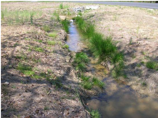
Photo Point 11. Upstream from ~SREV 24+00 to Curve C-20
