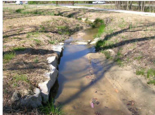
Photo Point 12. Upstream Grade Control Vane (SREV 25+00)
