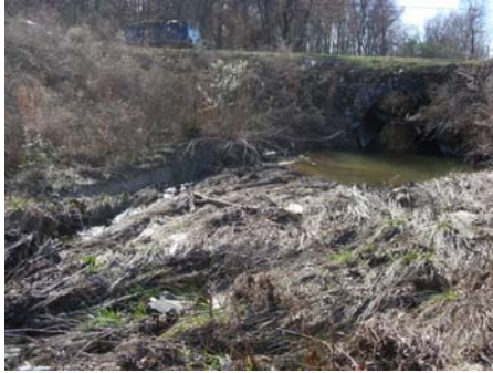
Photo 1: Representative fine sediment aggradation and bar formation problem area (Station No. 10+08; view upstream 2-20-2008).
